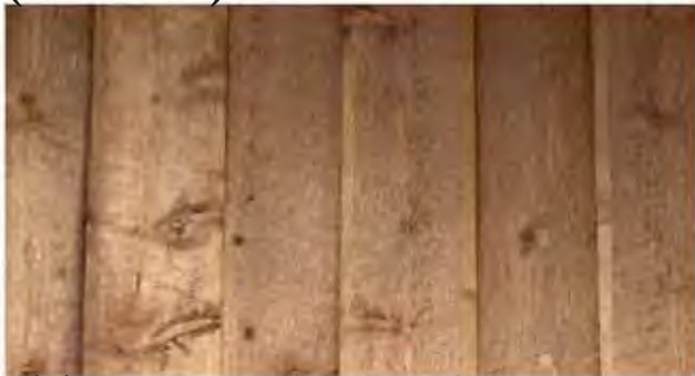
STAINED WOOD SIDING AND TRIM
