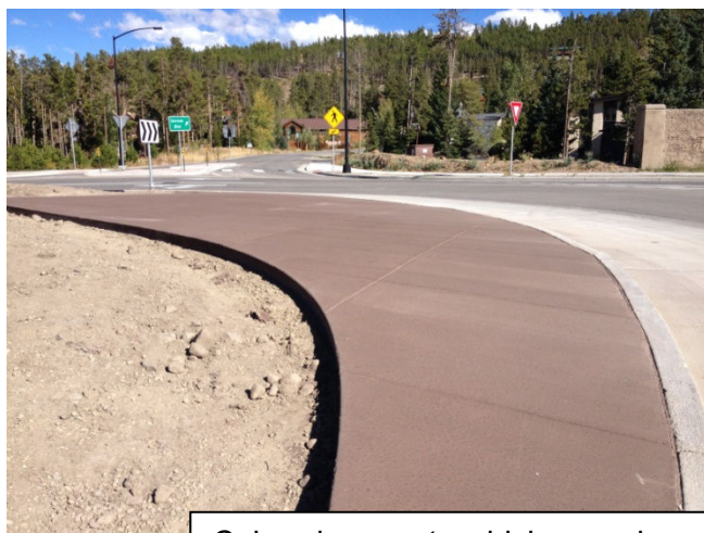
Colored concrete which was placed this week in the roundabout. The concrete matches the color and appearance of the Median "A" Concrete.
