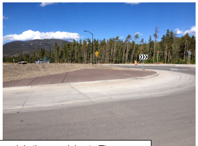
Colored concrete which was placed this week in the roundabout. The concrete matches the color and appearance of the Median "A" Concrete.
