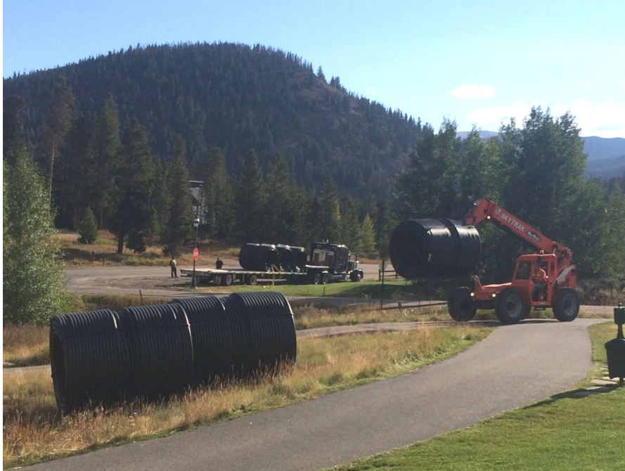
Taking delivery of 2000' rolls of 2" HDPE pipe.
