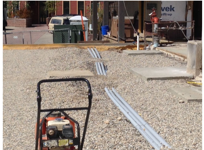
Electrical conduit is ready for inspection.
