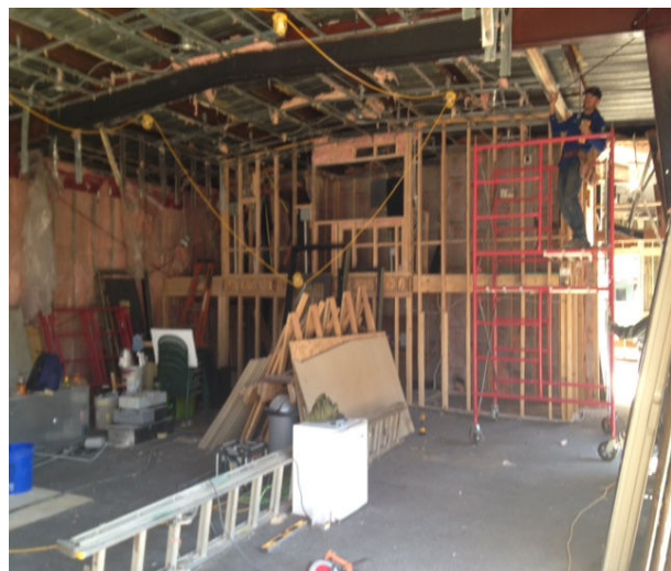
Framing for the expanded control room and mechanical space.
