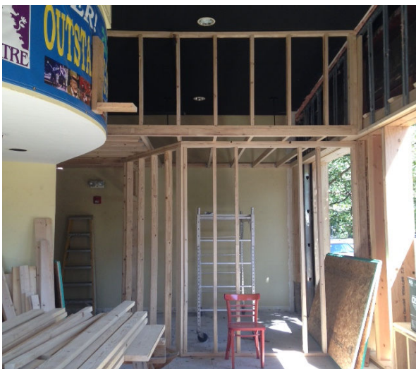
Framing for the new ticket booth.
