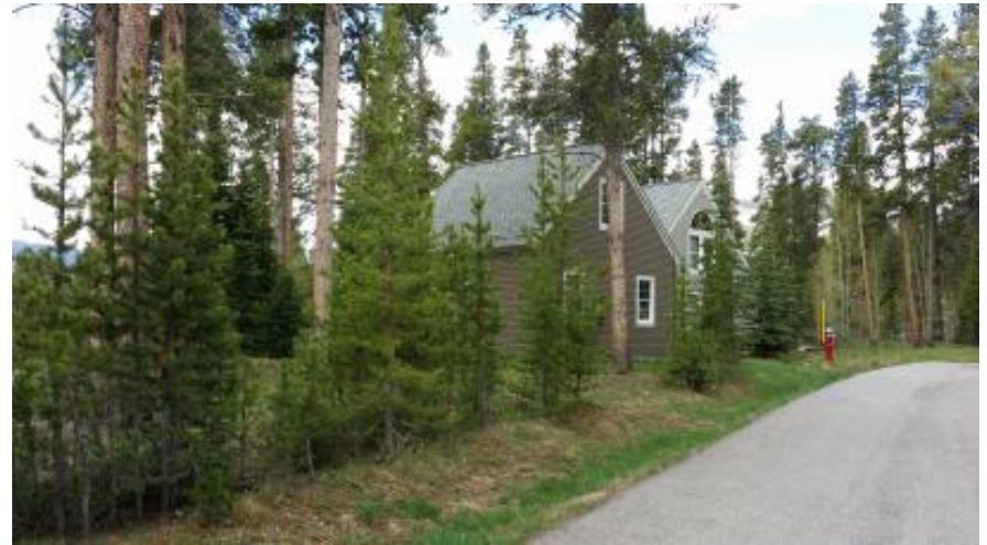
VIEW D – GARAGE FROM FAR PROPERTY CORNER
