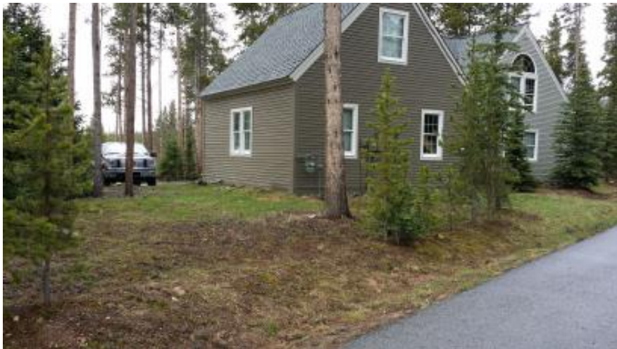
VIEW E – EXISTING GARAGE, LOCATION OF PROPOSED ADDITION
