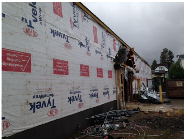
Exterior siding has been removed from the south side.
