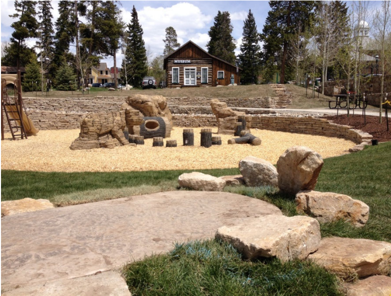
Concrete sculpture base for “Tom’s Baby”, which will be installed in fall of 2015.
