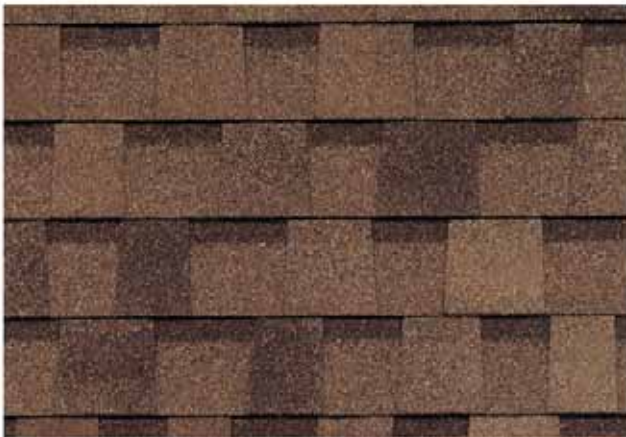
ASPHALT SHINGLES ROOFING
