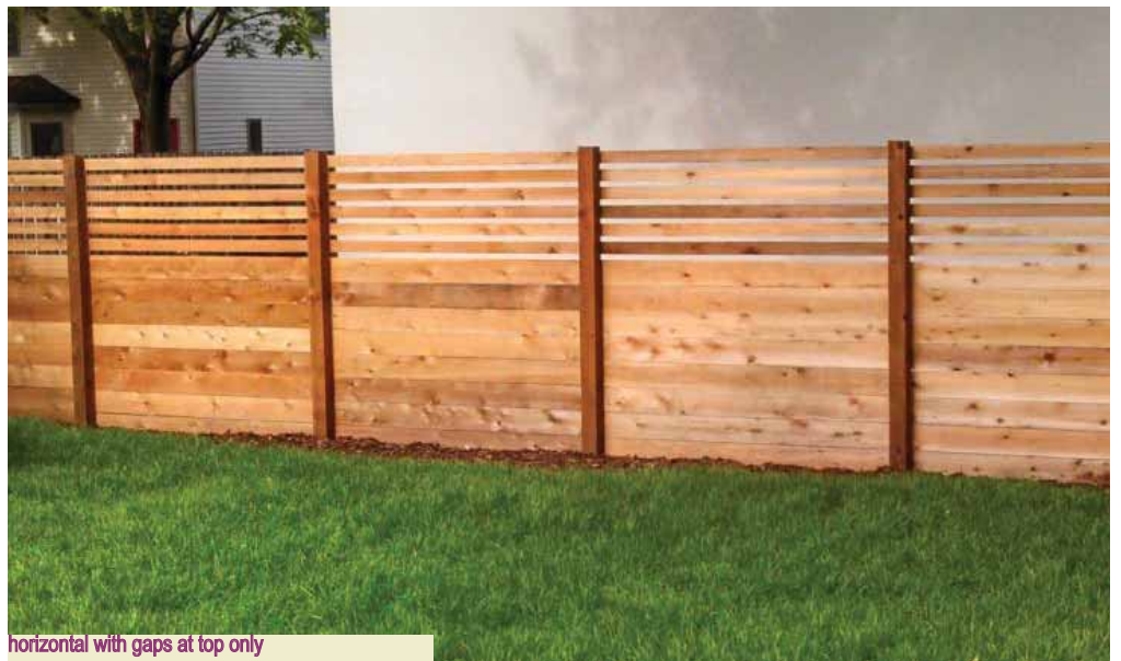
horizontal with gaps at top only
