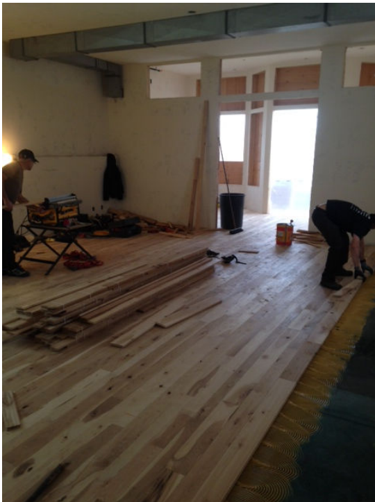
First floor studio looking west.
