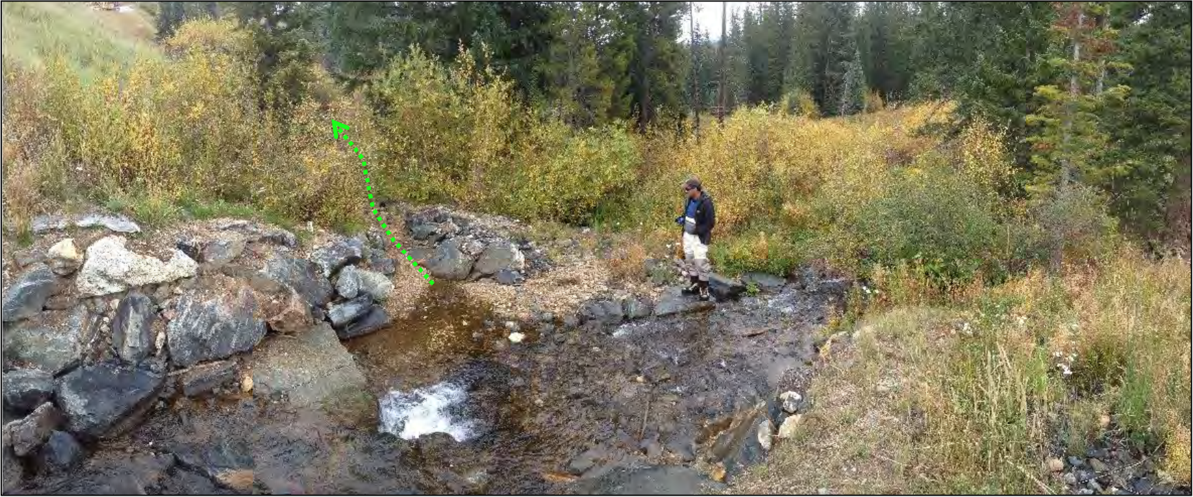
Photo C4a. This photo shows where the lateral channel (green arrow) splits off from Boreas Creek just downstream from a boulder energy dissipation structure.
