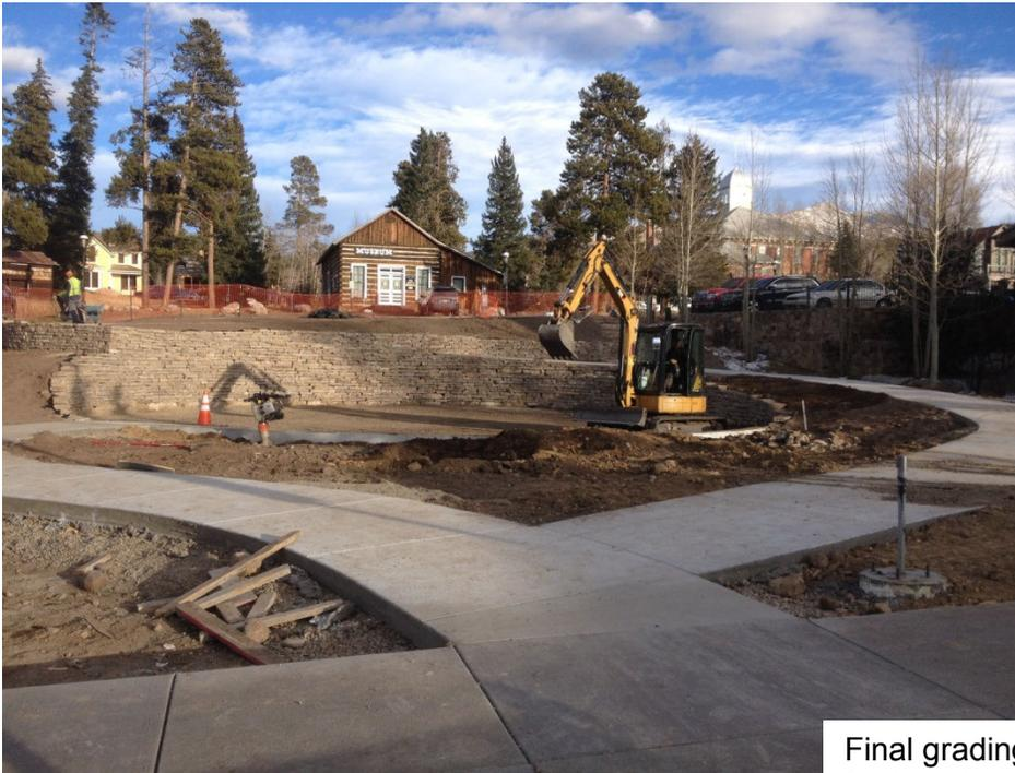
Final grading operations are being completed for the playground area. Next year, wood fiber will be placed inside the play area and playground equipment will be installed.
