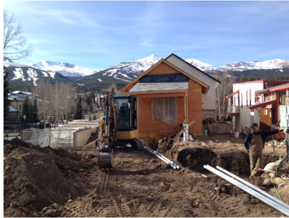
Electricians work on installing conduit to the building.
