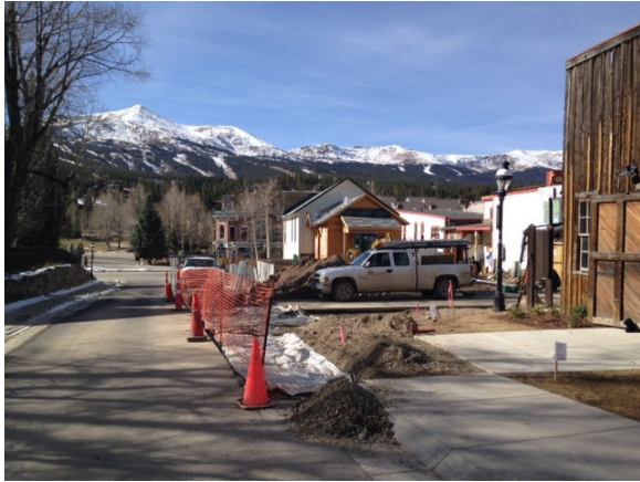
Curb and gutter is prepped for concrete.
