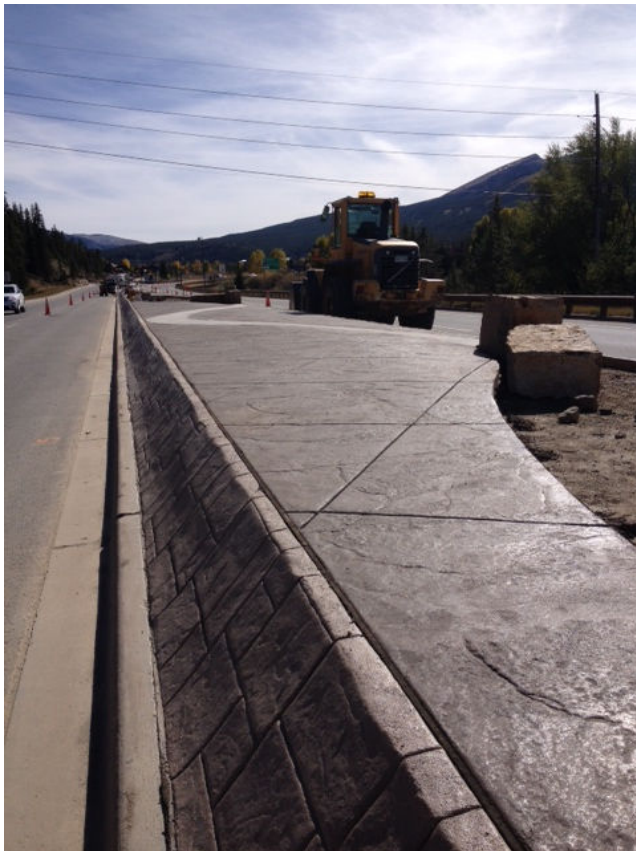
New stamped concrete and splash guard along the median.
