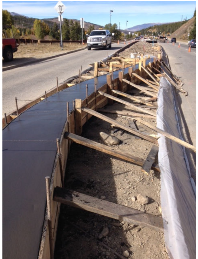
Concrete “ski track” being formed and poured.
