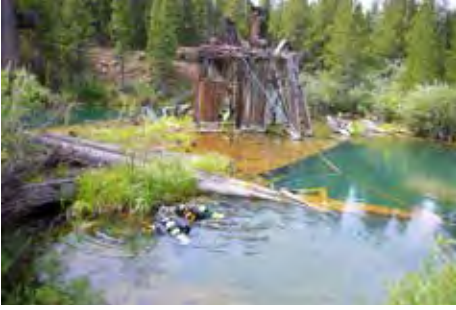
Divers evaluating underwater superstructure components
