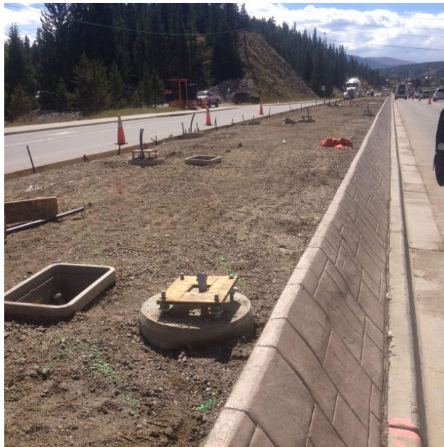
Concrete bases for poles which will display banners and flower baskets.
