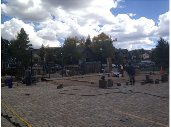
The concrete pavers are installed in the “Ridge Street Arts Square”
