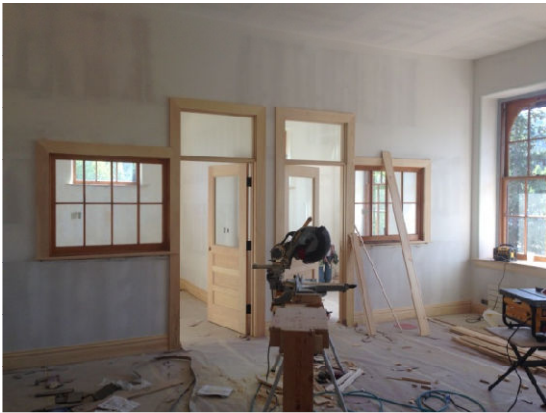
Installation of new doors and trim in the non-profit spaces is shown to the left. Placement of new tile flooring in the restrooms is shown below.
