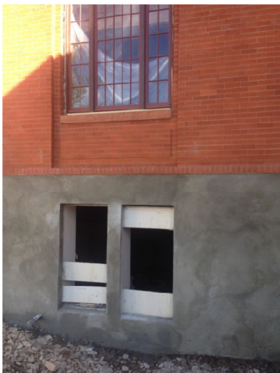
Left: New parge coat being placed on the building foundation.
