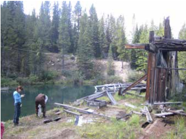
Anthony & Associates examining the condition of the deck of the Dredge.
