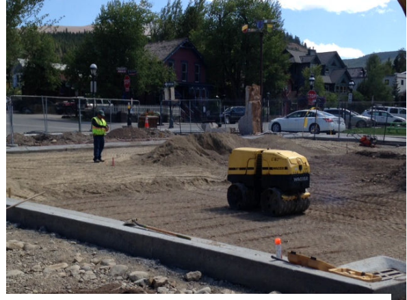
The parking lot sub-grade is compacted and prepared for new pavers.
