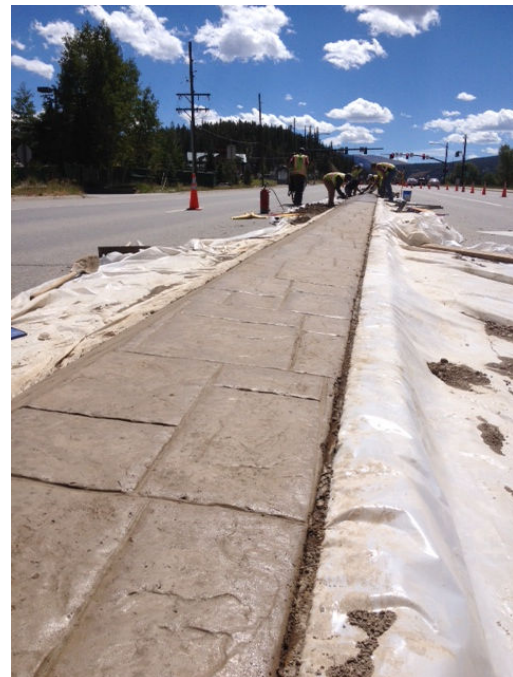
Colored concrete is being poured and stamped in the Highway 9 Median.
