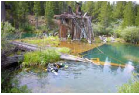
Divers evaluating underwater superstructure components
