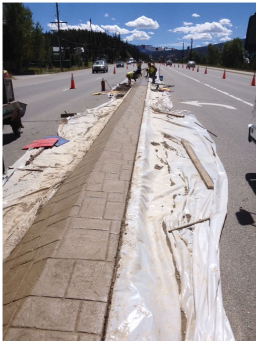
Colored concrete is being poured and stamped in the Highway 9 Median.
