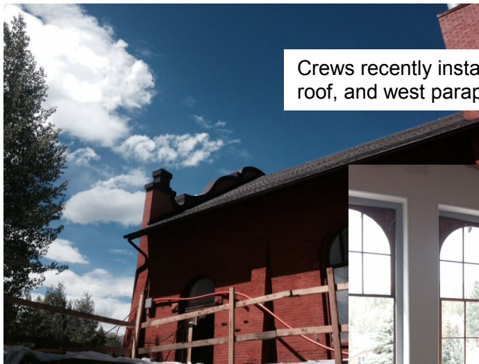
Work began this week with the installation of the refurbished historic windows in the 1909 building (Archive room pictured).
