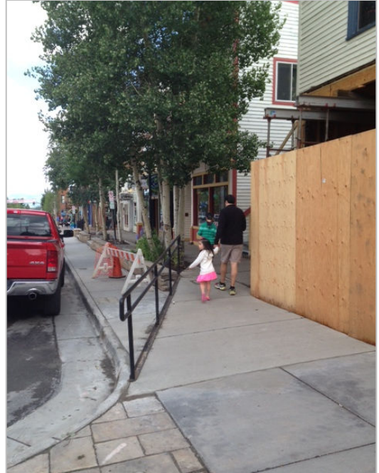
A temporary sidewalk directs pedestrians to neighboring businesses.
