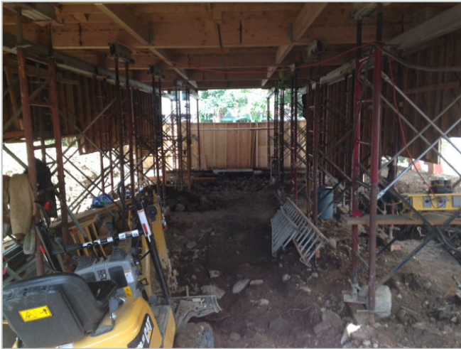
The view looking under the building to Main Street.
