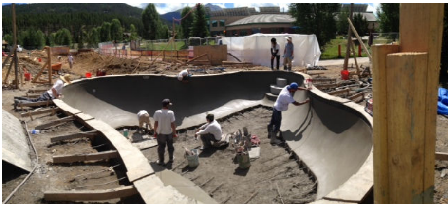
The crew is finishing the fresh concrete in the beginner bowl.
