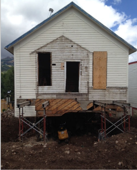
The building is lifted to build a new foundation.
