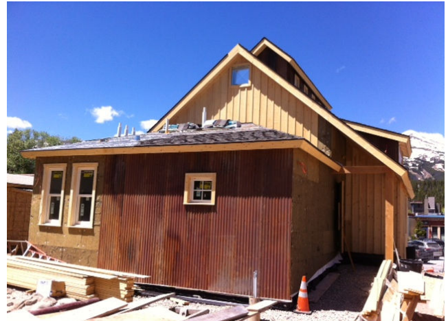
The monitor and east elevation of the Ceramics building are finished with corrugated metal siding.
