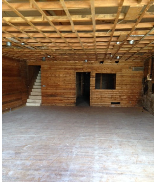
View of the historic interior wall on the first floor.
