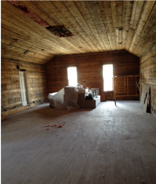
Second floor of the Old Masonic Hall.
