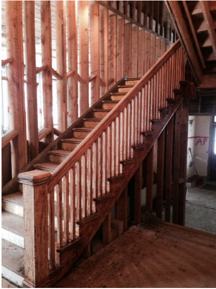
Existing Stair Railing in 1909 (left)
