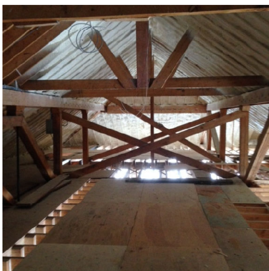
Installation of new insulation in the 1909 attic.
