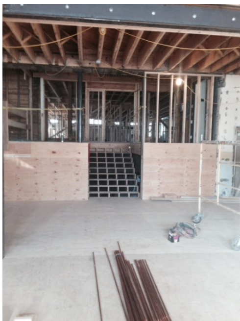
New stairs to Library main level.
