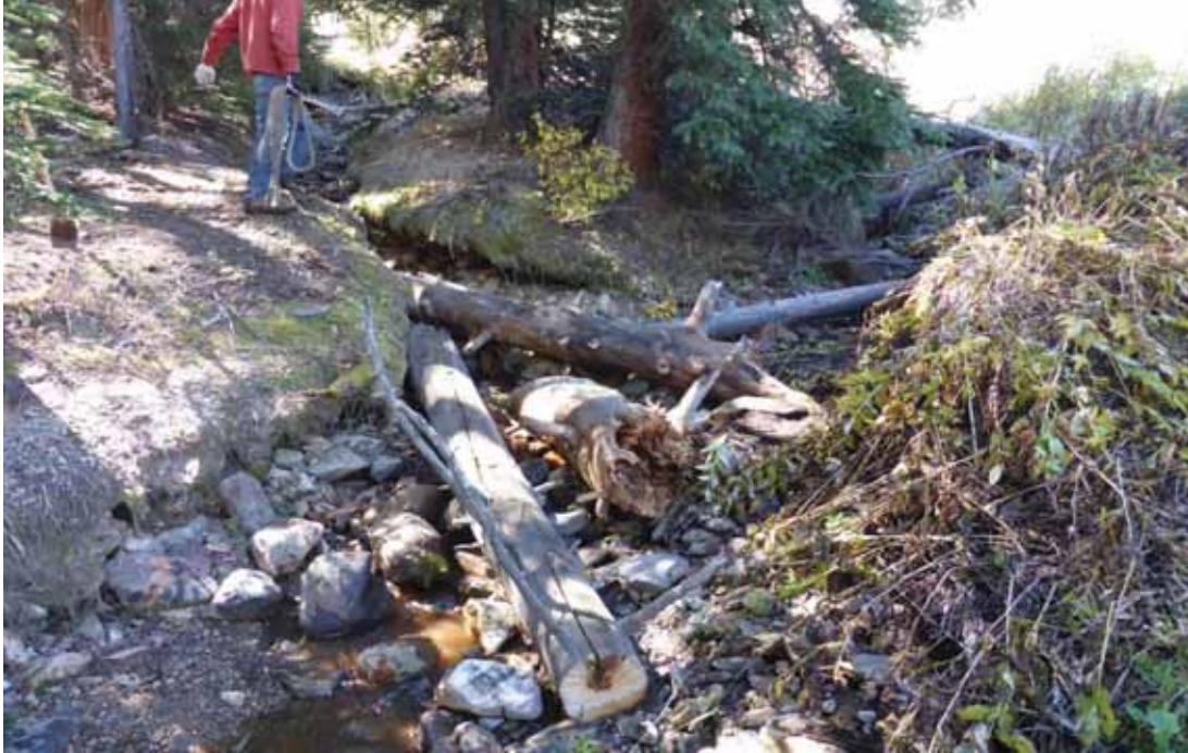
Photo 12. Same area but looking downstream on outlet of incised and narrow channel section. Large log structures on left side where a side channel enters from now active beaver ponds placed to prevent headcut from pond outflow.
