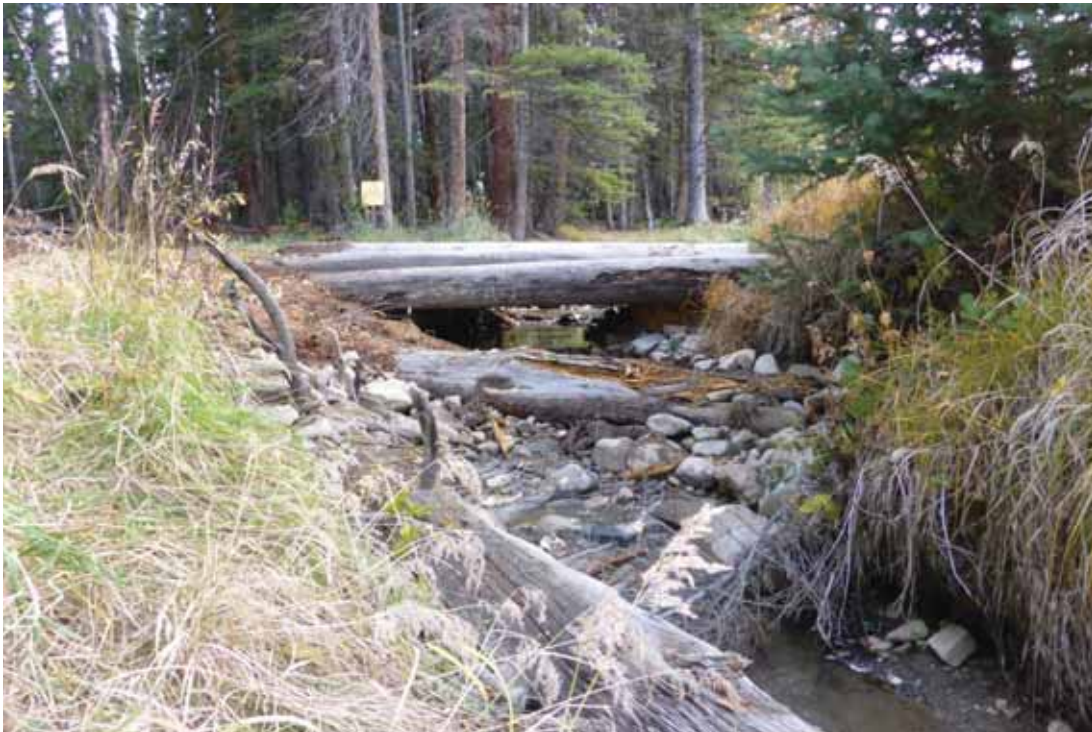
Photo 16. Upstream portion of project, logs and pitrun placed to fill channel, raise grade and slow velocity. Woody debris supported by pitrun will prevent further channel erosion.
