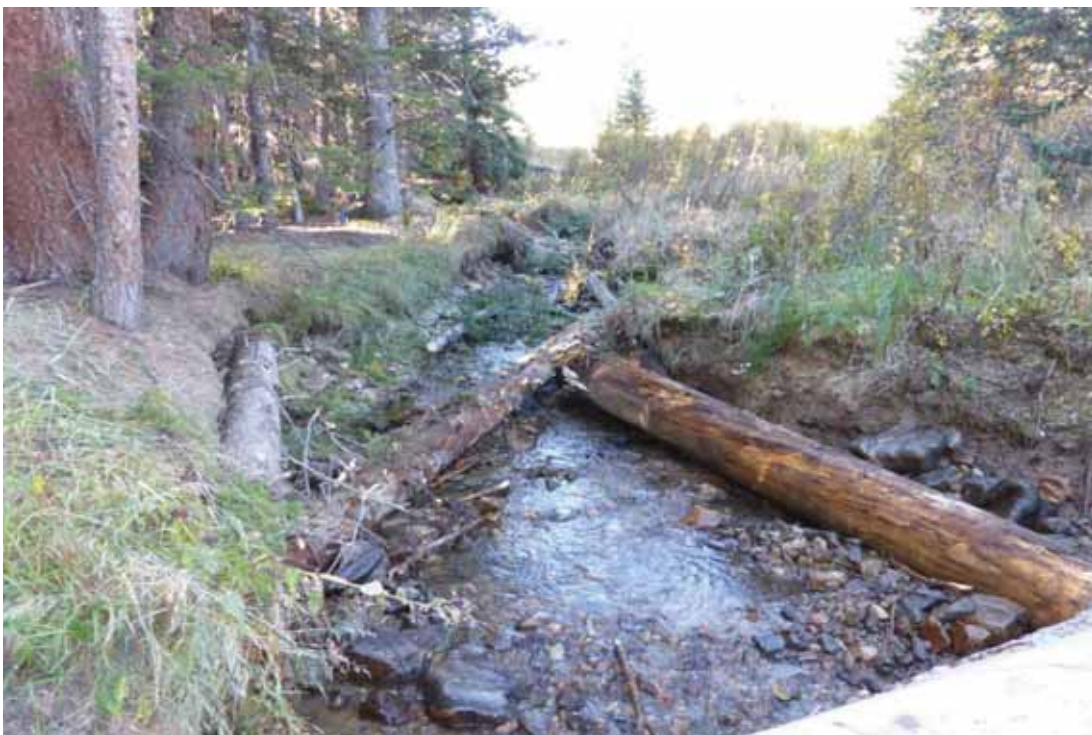
Photo 8. Starting to build upstream V-Log structure.
