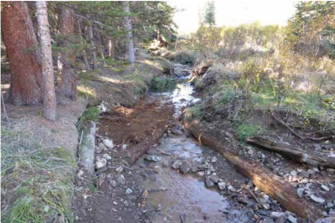
Photo 10. Structure complete. Topsoil added and left exposed on lateral bar to allow sediment (fines) to wash downstream to help seal next structure downstream.
