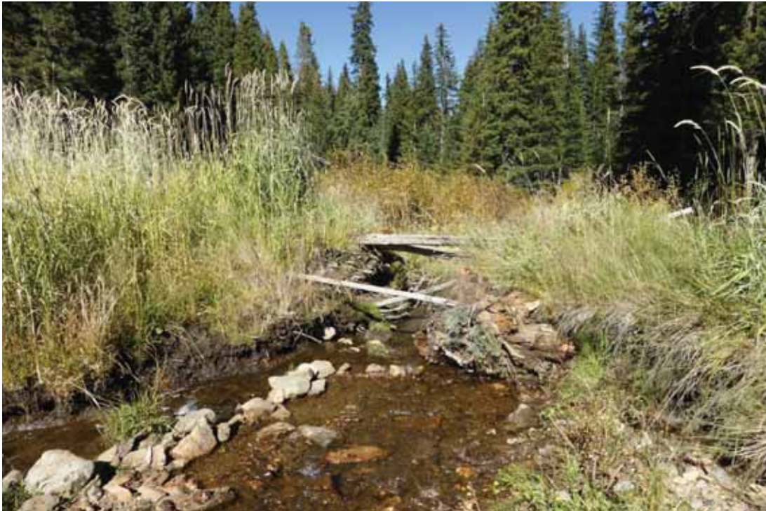
Photo 2. Starting on dam reconstruction at incision using logs, pitrun and whole live willows.
