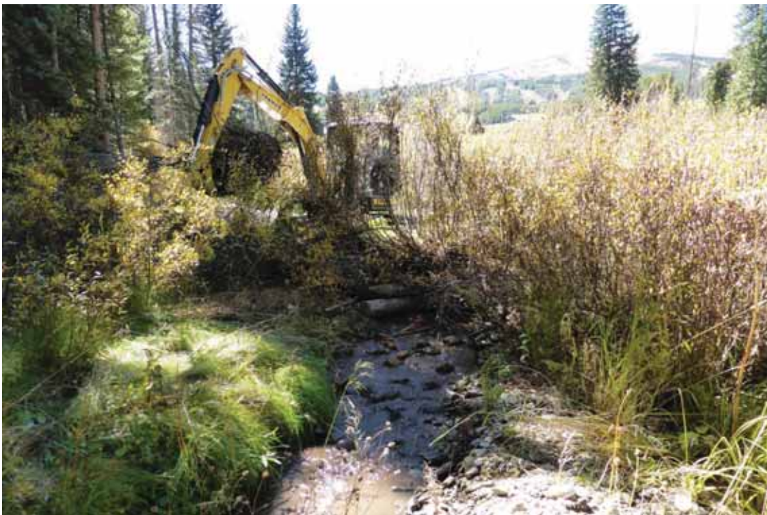
Photo 6. Reconstructing second dam downstream. Adding whole live willows onto of base constructed with large logs and pit run.
