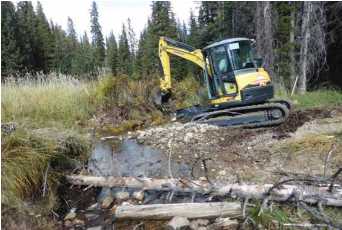
Photo 4. Downstream side of same dam rebuild. Note logs mixed with pitrun for added stability.
