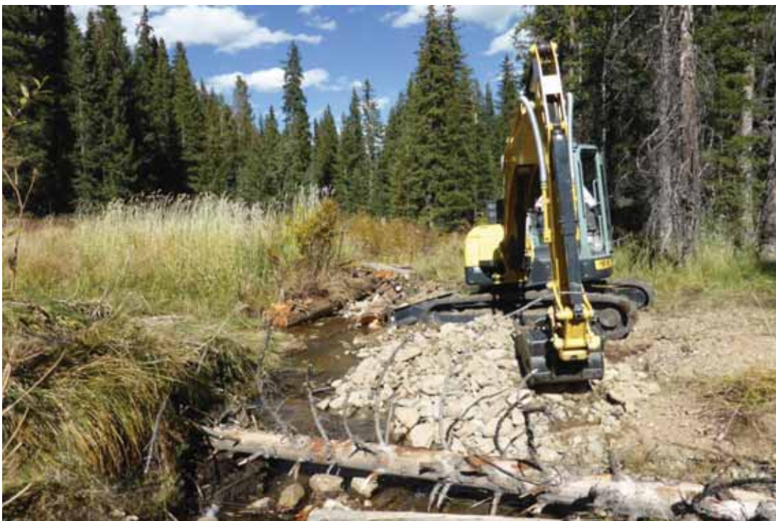
Photo 2. Starting on dam reconstruction at incision using logs, pitrun and whole live willows.
