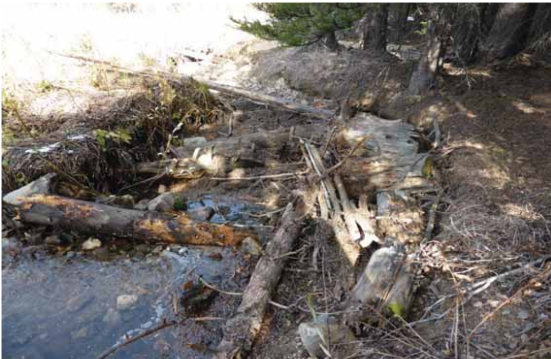
Photo 16. Upstream portion of project, logs and pitrun placed to fill channel, raise grade and slow velocity. Woody debris supported by pitrun will prevent further channel erosion.
