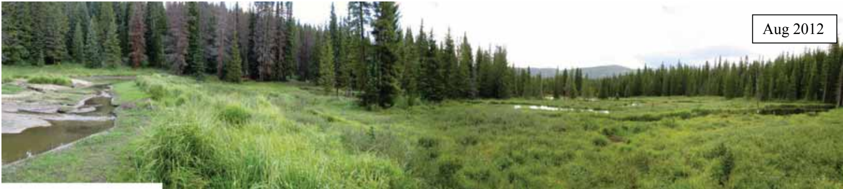
Photo C19. Photopoint 23, before and after restoration of the reset pond. The full pond elevates the local water table, and it spills along the width of the dam crest supplying water to a system of distributary channels downstream of the dam. The channels are in the vegetation towards the right foreground of these photos, and they feed ponds in the right background.
