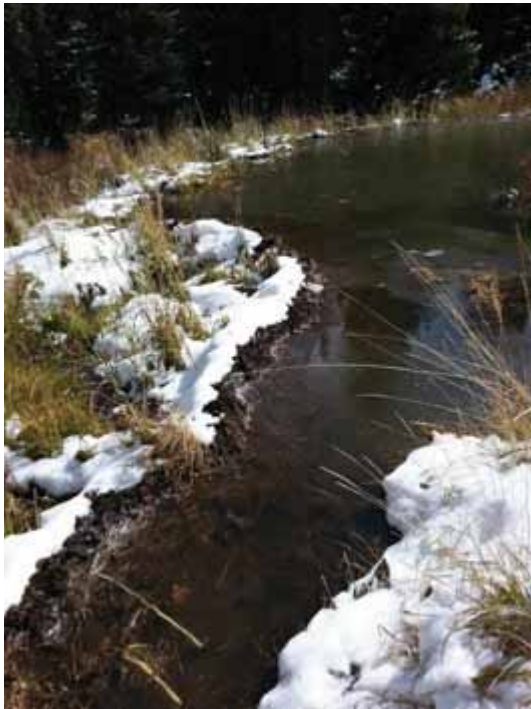
Photo 2.7: Close-up of dam work at top of Gulch
