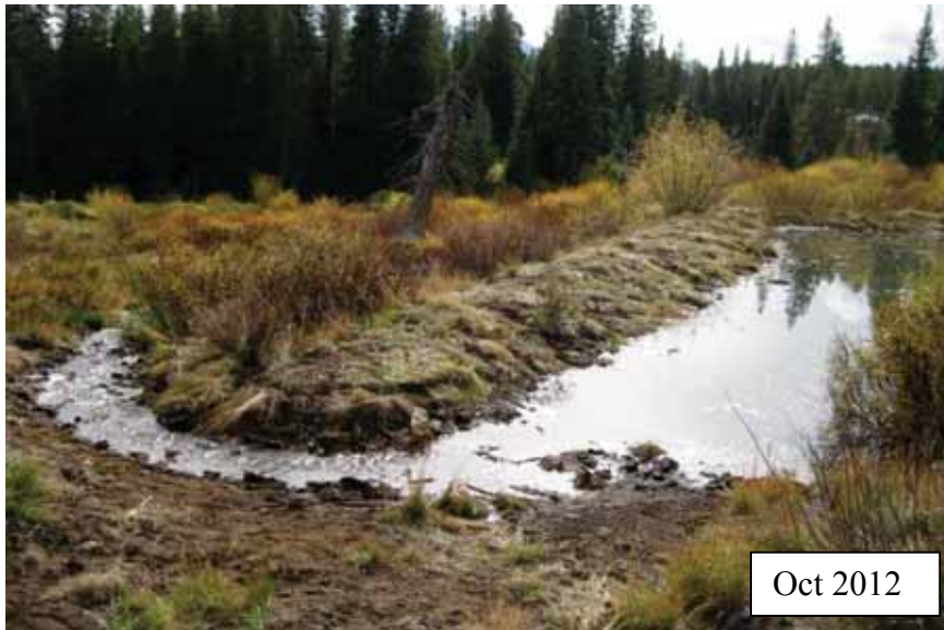
Photo C12. These photos show the west end of the spreader pond as constructed in October 2012 (upper photo) and on August 29, 2013, soon after beavers reoccupied the area (lower photo). In 2013, beavers plugged the constructed spillway channel which allowed the pond to function fully for spreading water. In the lower photo, the pond is full to the crest of the dam (foreground and left edge) which is being maintained by the beavers (the rings on the pond are from a beaver packing mud on the dam face). The full pond spreads water among a number of distributary channels downstream.
