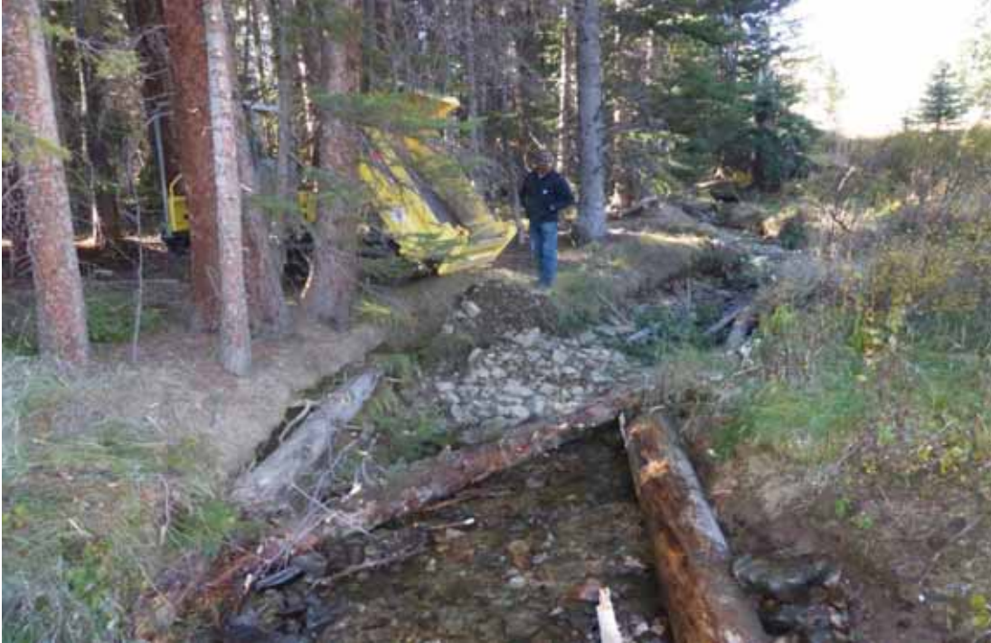
Photo 10. Structure complete. Topsoil added and left exposed on lateral bar to allow sediment (fines) to wash downstream to help seal next structure downstream.
