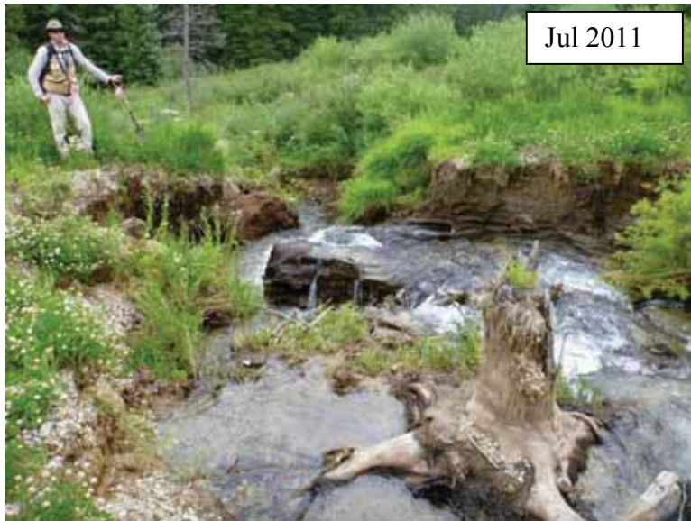
Photo C7. Photos of the incised Boreas Creek channel that had recently formed by erosion through the entire length of Upper CG, as seen in 2011.
