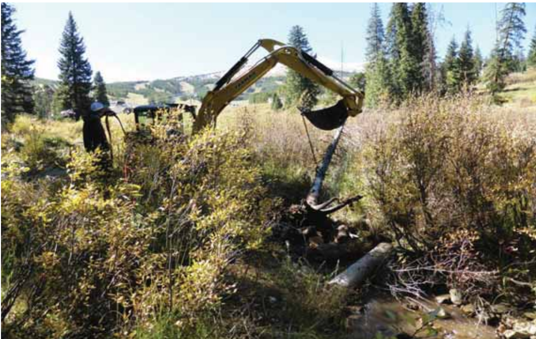
Photo 18. Log with root wad placement in lower dam rebuild. Chain used to maintain integrity of log. With the right operators, track hoe can sit right in wetland and channel with minimal disturbance.
