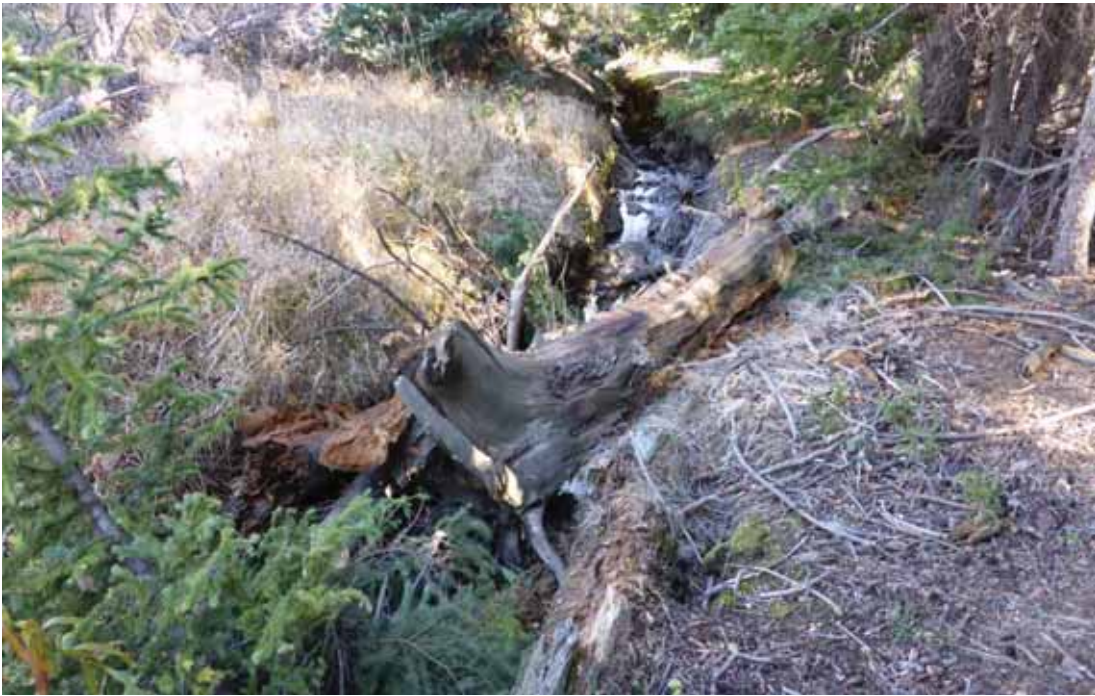
Photo 18. Log with root wad placement in lower dam rebuild. Chain used to maintain integrity of log. With the right operators, track hoe can sit right in wetland and channel with minimal disturbance.
