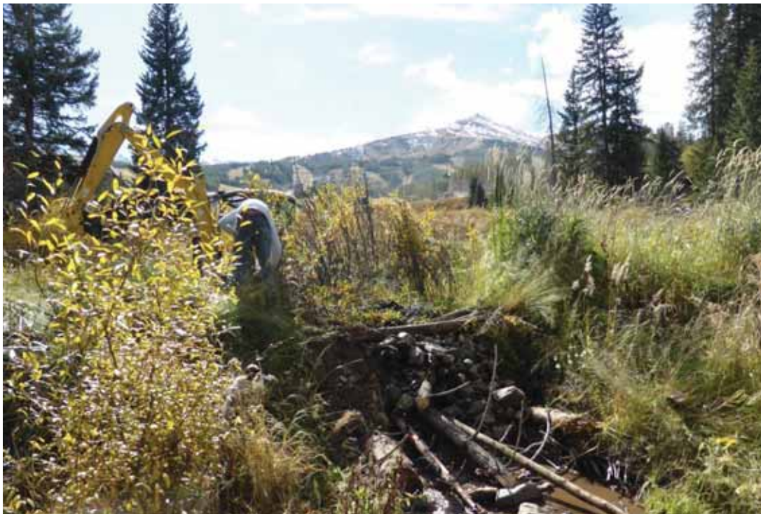
Photo 4. Downstream side of same dam rebuild. Note logs mixed with pitrun for added stability.
