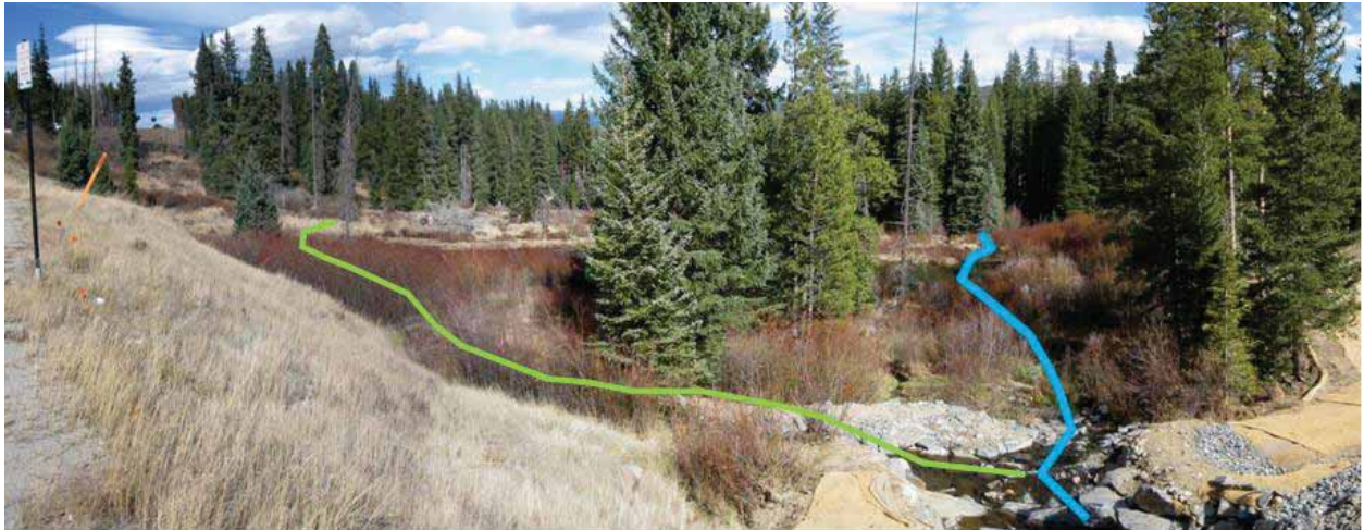
Photo C8. One of the treatments aimed at improving water source and distribution was construction of a lateral distribution channel that draws water from just downstream of the Boreas Creek culvert to spread it northward along the toe of the road fill at the head of Upper CG. The upper photo and the lower right photo shows the alignment of the new channel (shown in green) and the main channel of Boreas Creek (shown in blue) just after construction in October, 2012. The lower right photo shows a segment of the new channel in August, 2013.
