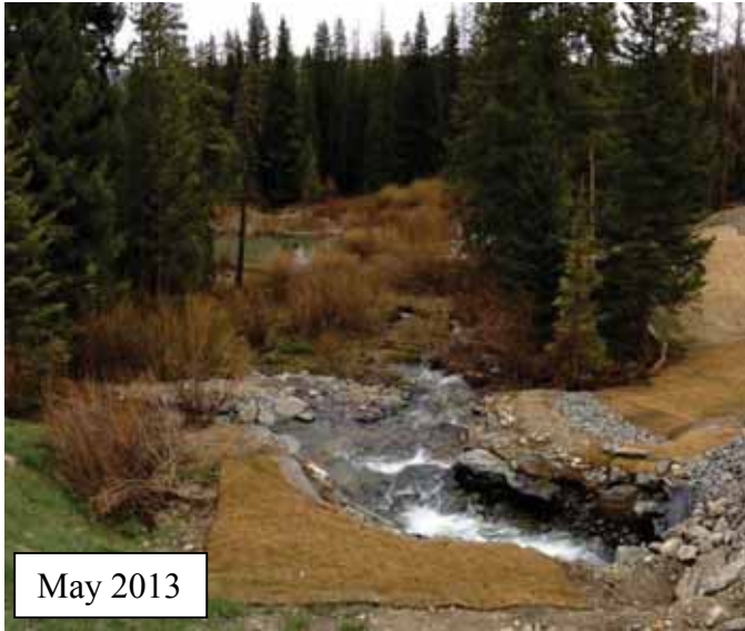
Photo C6b. Photopoint 3b, 2013. The Boreas Creek culvert outlet. The flows seen in the photo from May are typical of snowmelt runoff. The low in the September photo shows runoff from a small thunderstorm. Note the severe turbidity.
