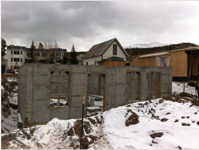
Foundation of the new ceramics studio.
