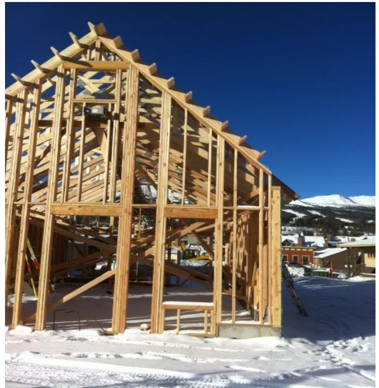
Framing of the new metal smithing studio.
