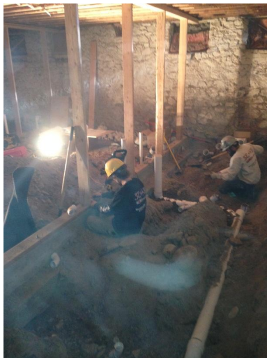
Rough-in plumbing for coffee shop and kitchen.
