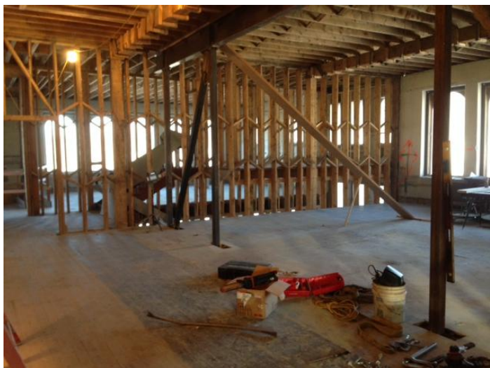
Historic framing and new steel structure in children's area.
