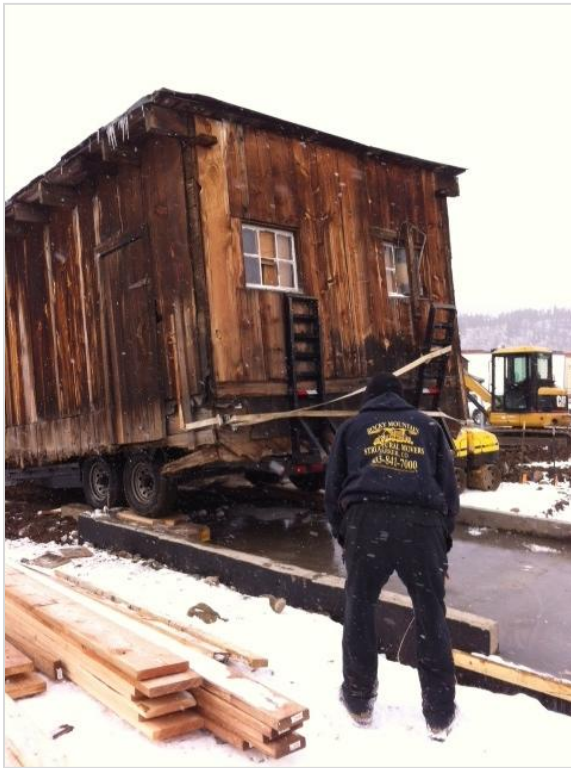
Moving the historic Little Red Shed to its new foundation.
