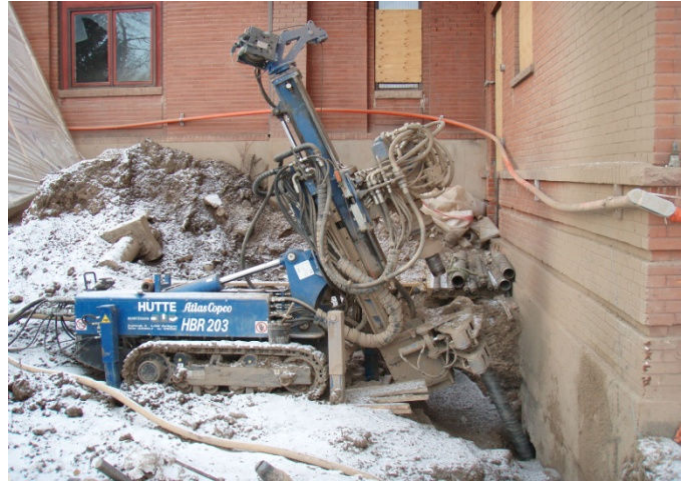
The installation of micro-piles at the existing building corners and interior walls adding additional strength to the existing foundations.
