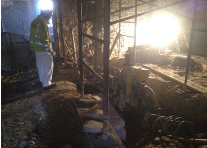
The installation of micro-piles at the existing building corners and interior walls adding additional strength to the existing foundations.
