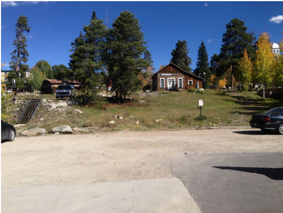
Figure 1 - Looking west across the proposed park site to the Edwin Carter Museum
