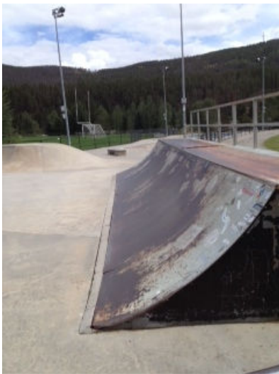
Metal quarter pipe box in street section
