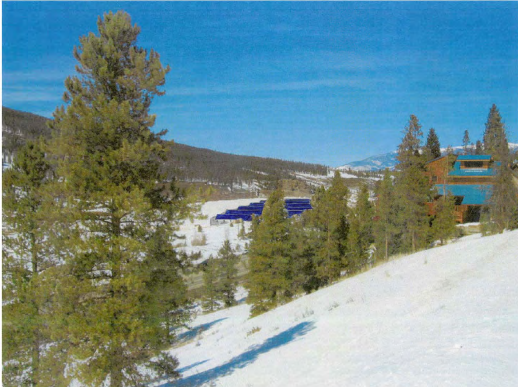
PHOTO E FRONT OF ARRAY VISIBLE
