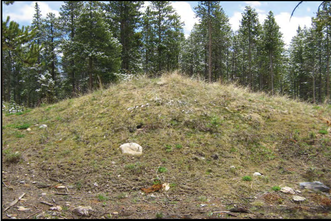
Photo 3: Example of waste rock consolidation area; work completed under VCUP program using CO Best Practices for Abandoned Mine Reclamation .
