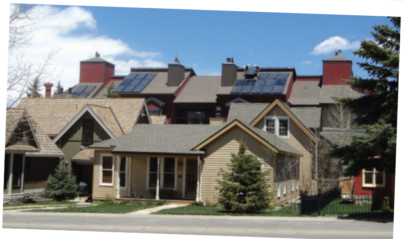
The solar thermal installation allowed each resident in the condominium complex to receive a $500 federal tax credit.
