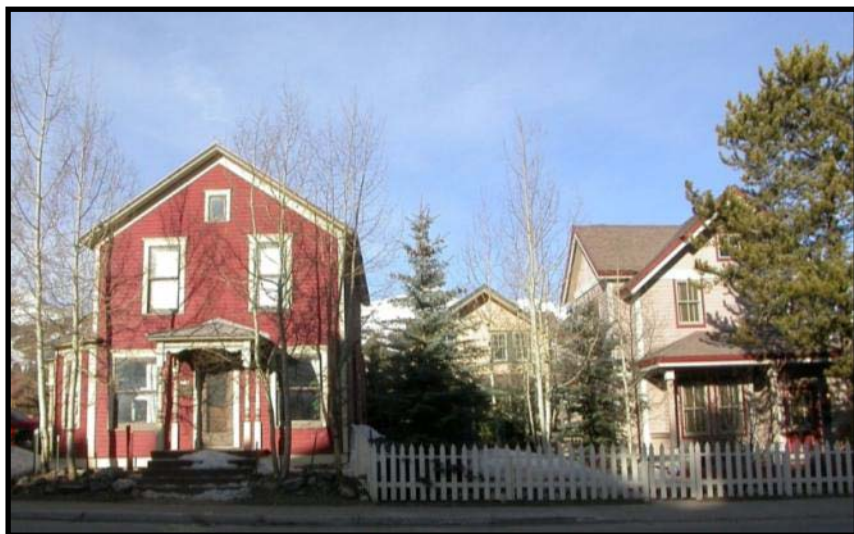
New commercial development should maintain a single family residential character. Future development should also convey the rhythm of the smaller historic lots wherever feasible.
