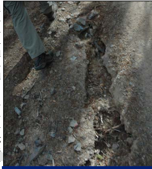
Trail damage resulting from unsustainable trail
