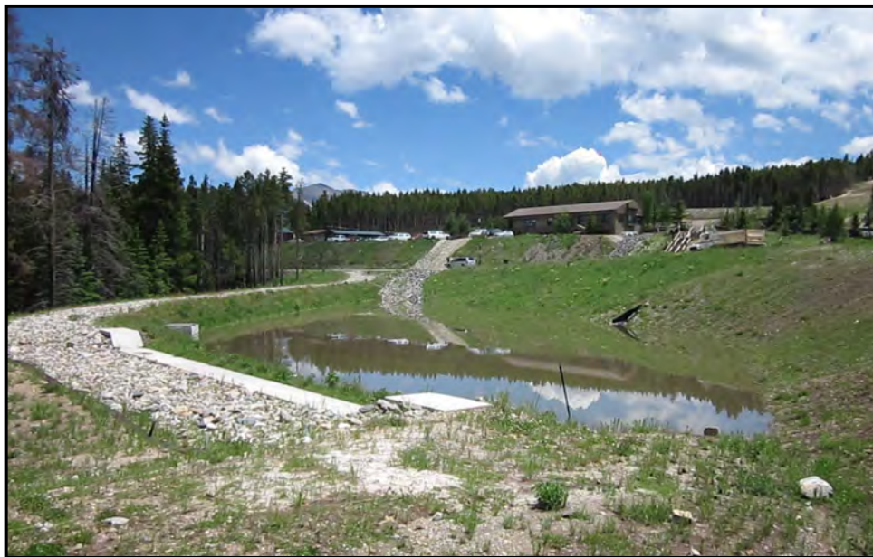
Photo 15. Surface runoff from some of the Peak 8 base area flows into this retention pond which held water for the length of the 2011 season.
