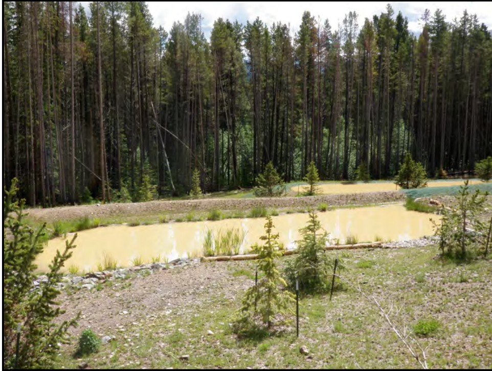
Photo 11. Water in detention ponds was often turbid long after storm events. Most of these ponds have surface water outlets to Peak 7 SS or Upper CG wetlands. While some of the suspended sediments did settle out in ponds, outflows to CGP were regularly high in turbidity. Water quality stressors of this type tended to be limited to the wetlands at the upper edge of these units.
