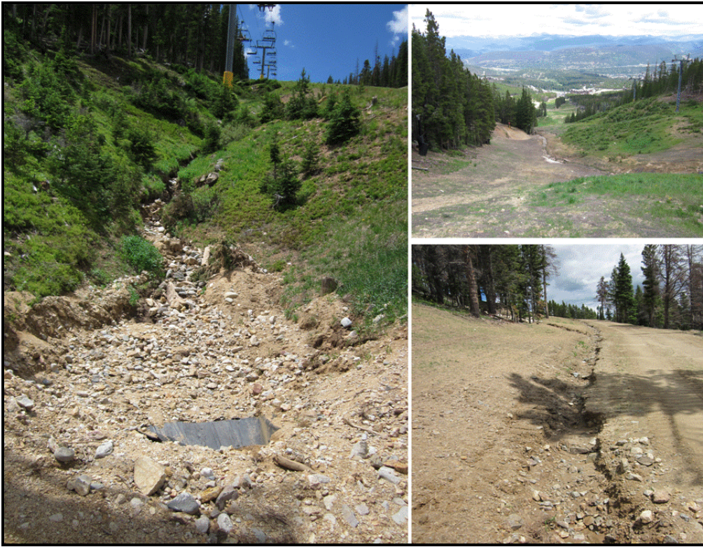
Photo 24. The source watershed for Upper CG is entirely within a ski area. There are many signs which indicate that activities within the watershed have an impact on the sediment regime.
