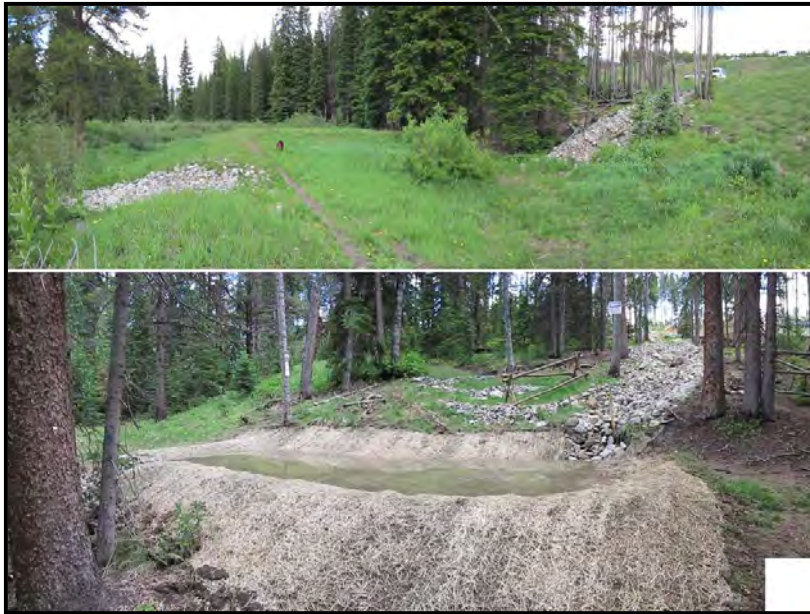
Photo 22. In addition to the main Peak 8 detention pond, two other primary storm drainage-ways enter CGP on the south arm of Upper CG. The Admin. drainage/detention pond (upper photo) was never observed to hold water during the 2011 season.
