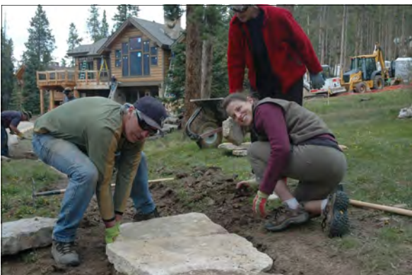
Trail Maintenance Project
