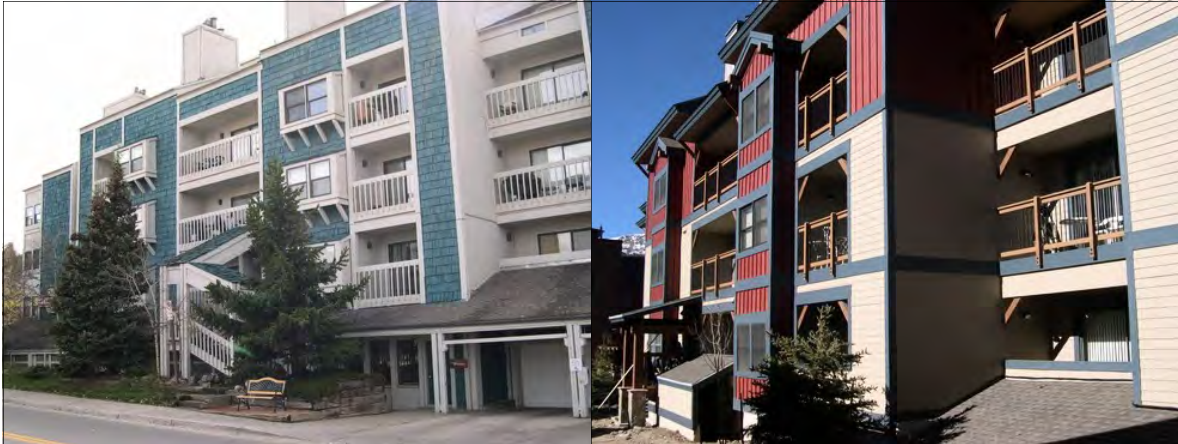
Before and after photos from a condominium renovation
