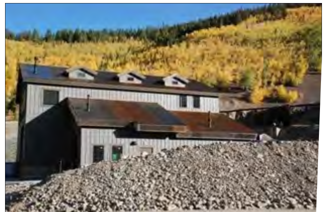
Wellington Oro Water Treatment Plant
