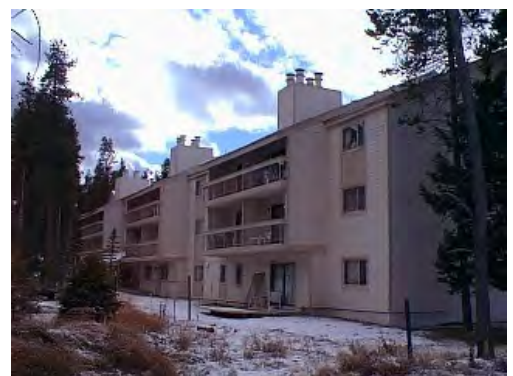
Typical Older Multi-family Development
