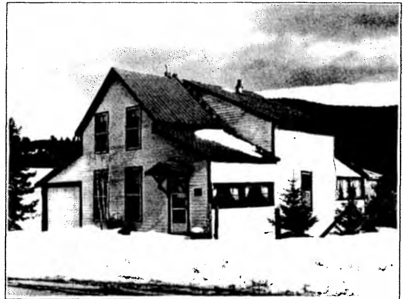
After rehabilitation, the historic material is visible and the historic integrity is enhanced.
