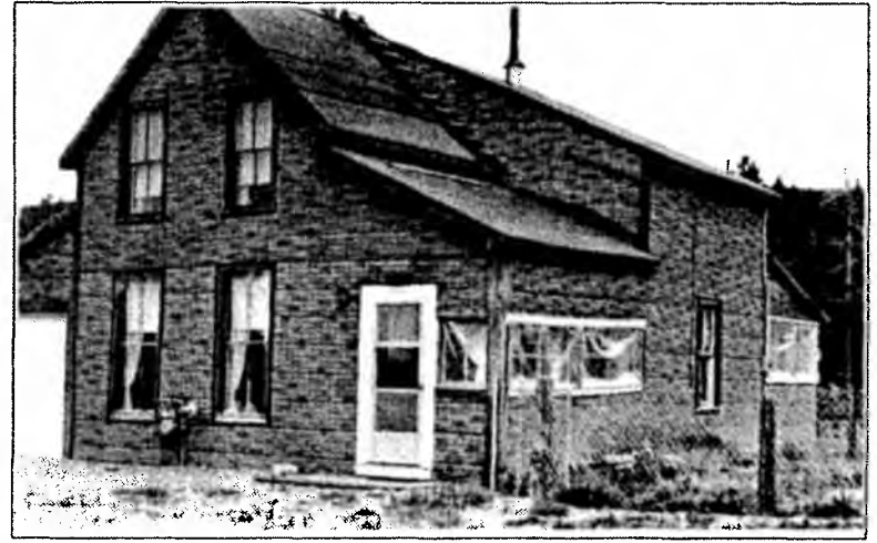
This photo of the Tillet House taken in 1978 shows an imitation brick siding that obscured the historic clapboard and diminished the integrity of the structure.
