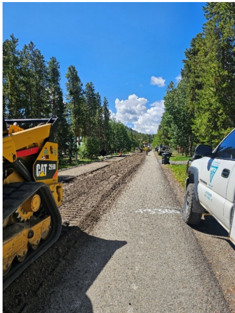
Photos of full depth reclamation and grading along Silver Circle.
