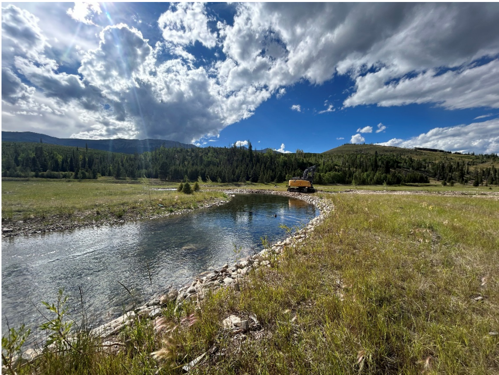
View of the bank repair looking west.
