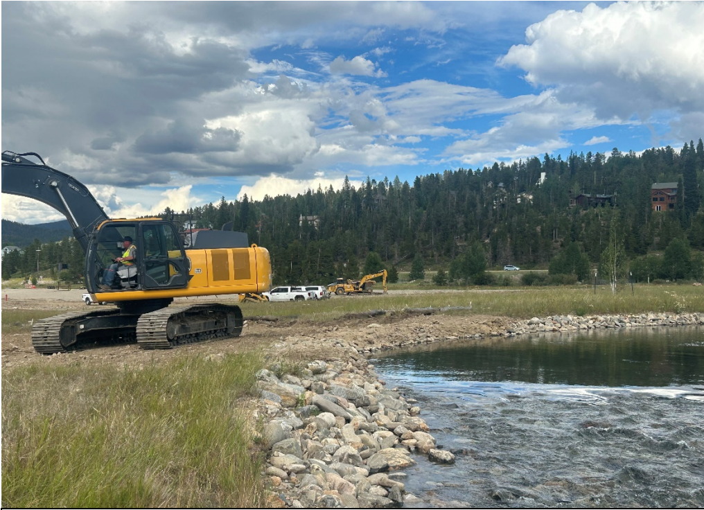
Material is replaced at an upstream bank.
