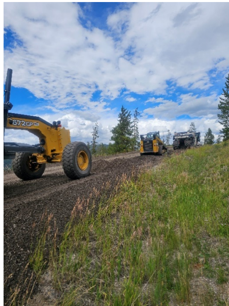
Photos of full depth reclamation and grading along Silver Circle.
