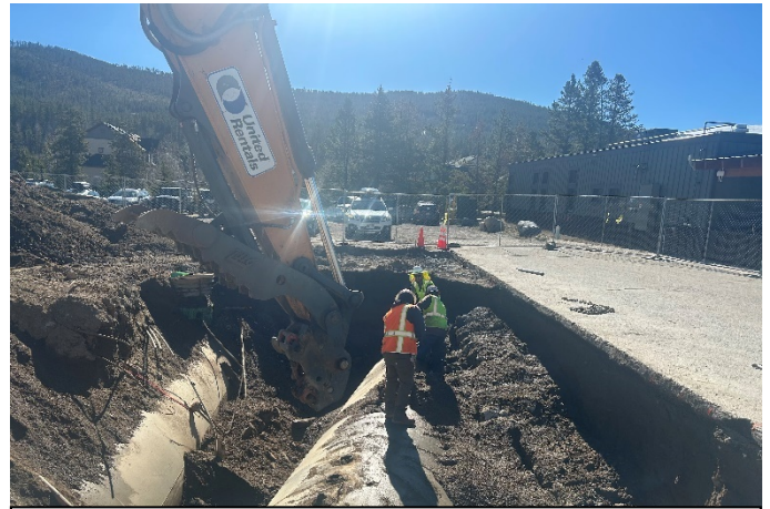
Crews work to expose the existing underground storage tanks.
