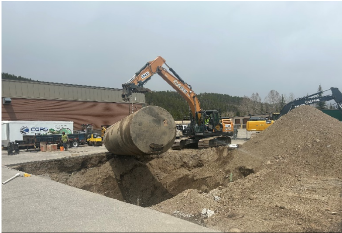
The existing underground storage tanks are removed from the excavation.
