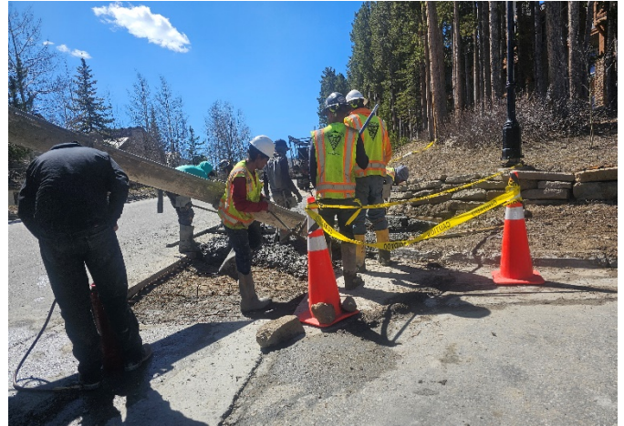
Concrete replacement at Snowflake Drive and King’s Crown intersection.
