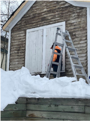
Figure 2. Exposed historic horizontal painted wood lap siding.
