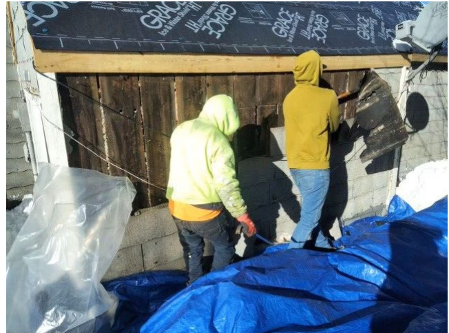
Figure 3. Exposed historic vertical wood siding with natural stain.
