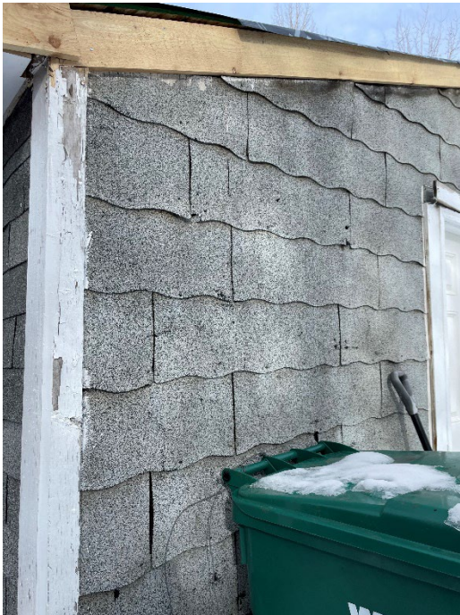
Figure 4. Detail view of scallop edged asphalt shingles.
