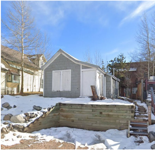
Figure 1. Structure prior to removal of asphalt shingle siding.
