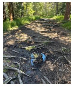
Turnpike removal will generate approximately 30 cubic yards (CY) of 3/8" crusher fines to be re-purposed for surfacing approximately 850 LF of new trail enhancing long-term drainage in the flatter terrain (<10% sideslopes).
