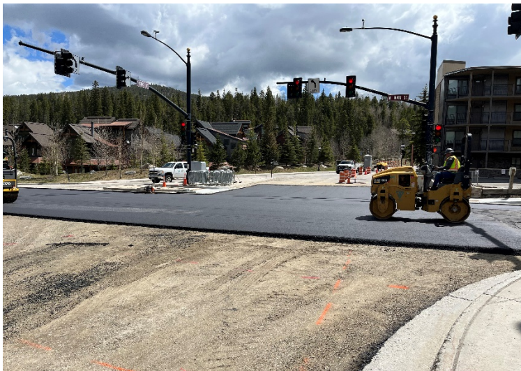
In the left photo above, asphalt is being repaved at the French Street intersection where a storm inlet and pipe were installed to improve drainage. In the right photo above, concrete sidewalk was replaced on Lincoln Ave.
