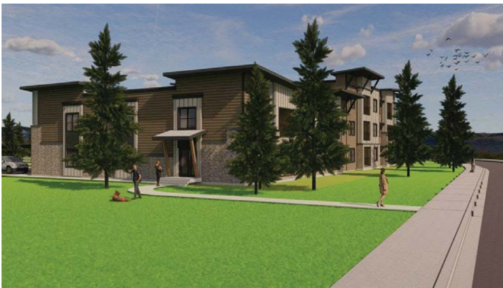
NORTHSIDE VIEW FROM AIRPORT ROAD
