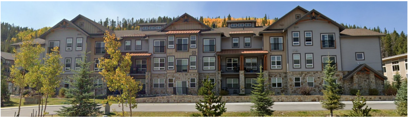
Image 8 (above): Pinewood II Employee Housing Apartments, looking West from Airport Rd.
