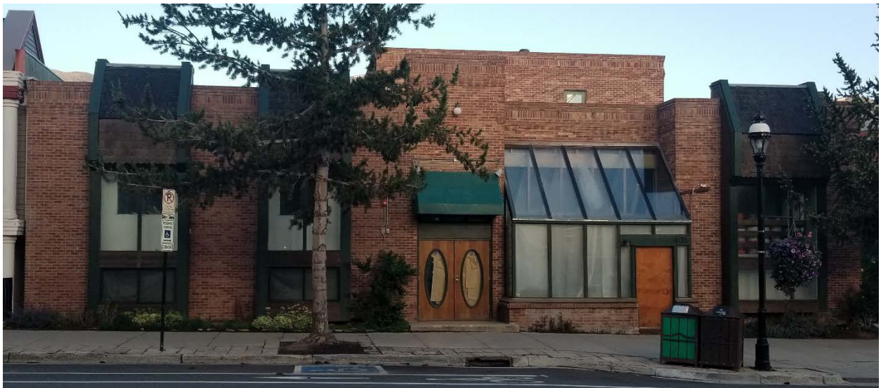
Image 1 (above): Photo of existing east elevation. Image 2 (below): Proposed east elevation modifications.
