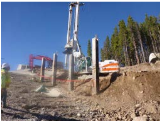
Drill rig installing shoring wall piles.
