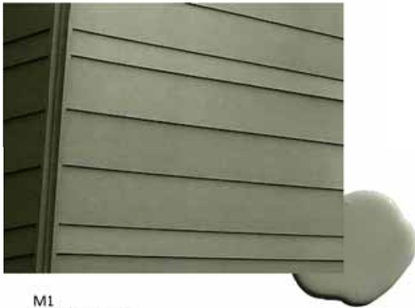
M1 PAVE CEMENT VERRING WITH LAP SIDING
