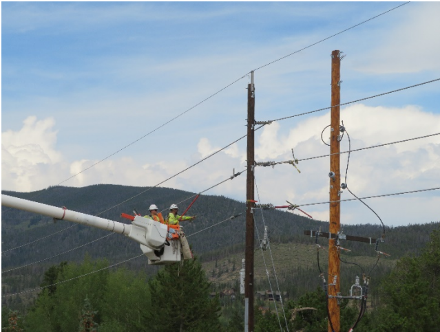
08/03/2020 – Removing Overhead Power
