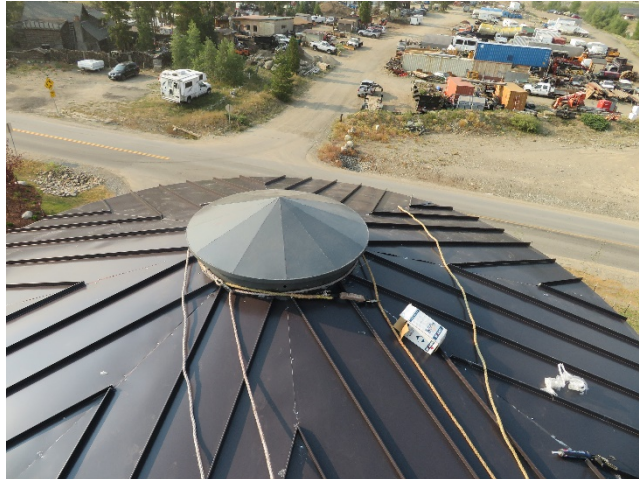
08/24/2020 – Blend Tank Metal Roofing
