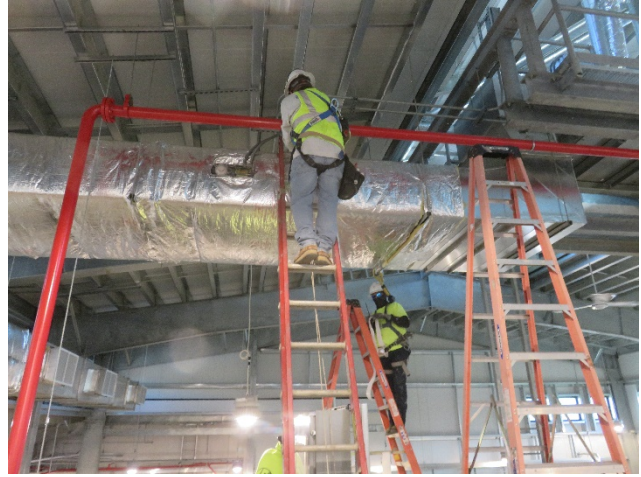
08/17/2020 – Ductwork Insulation
