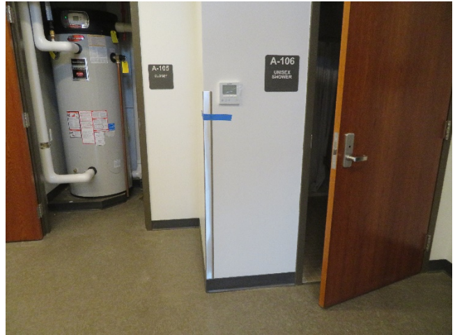
08/03/2020 – Administration Building Corner Guard
