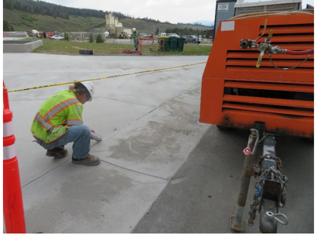
08/20/2020 – Concrete Pavement Caulking
