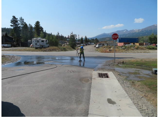
08/27/2020 – Pavement Pressure Washing
