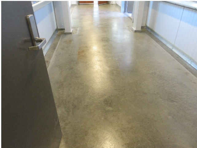
08/19/2020 – Covered Walkway Floor Sealant
