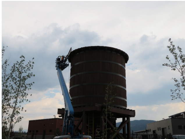
08/20/2020 – Blend Tank Shroud Metal Roofing
