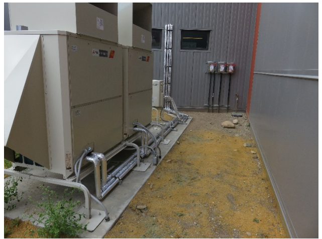
08/19/2020 – Refrigerant Piping Jacketing
