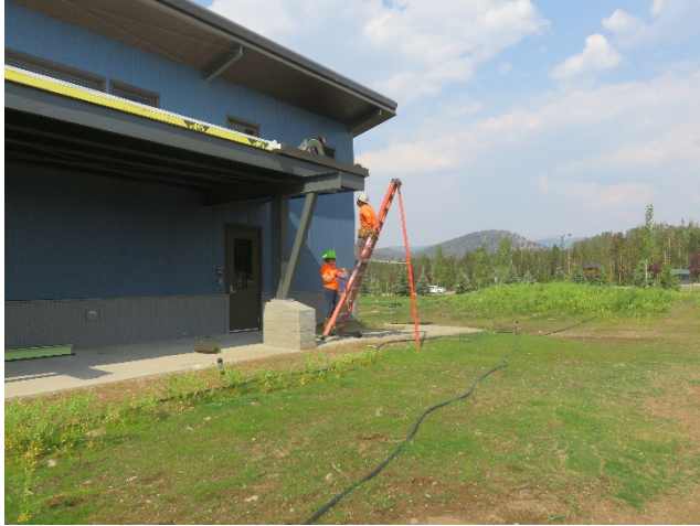
08/17/2020 - Administration Building South Canopy Roof
