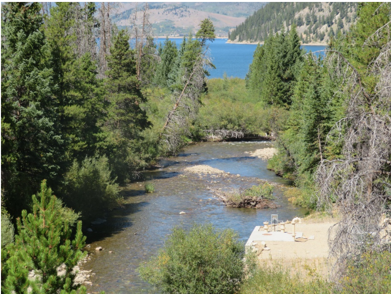
Raw Water Intake 09/03/2020
