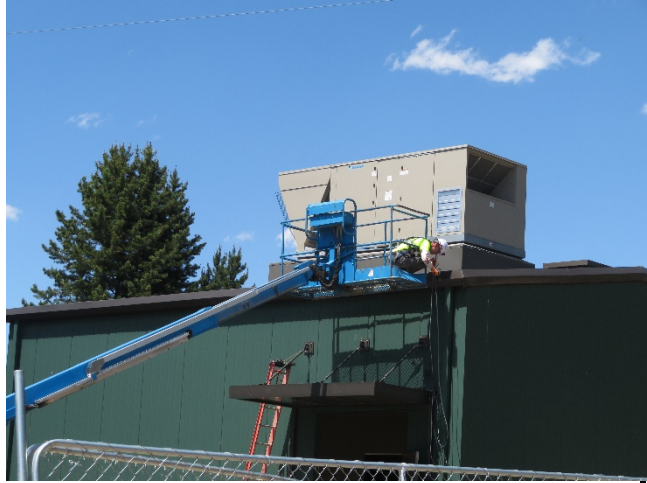
06/17/2020 – Raw Water Pump Station Heat Trace
