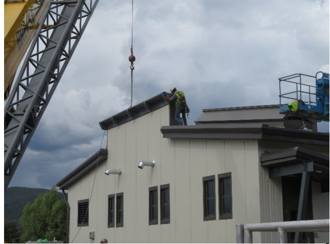
06/23/2020 – FWPS Store Front Top of Wall Trim
