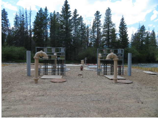
06/16/2020 - Valve Vaults Gooseneck Vents and Bollards.
