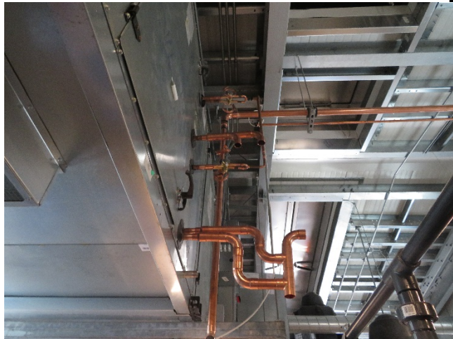
06/10/2020 – FWPS Refrigerant Piping
