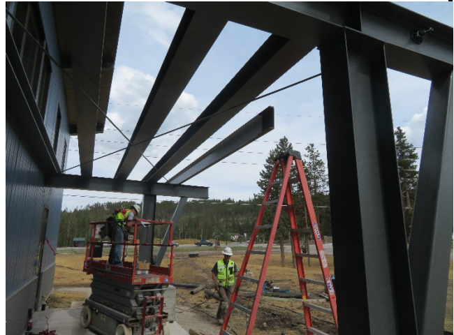
06/29/2020 - Administration Building South Canopy Roof
