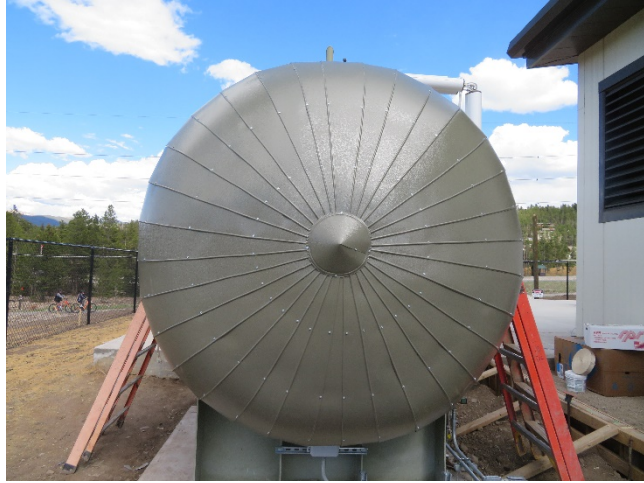
06/11/2020 - FWPS Surge Tank Insulation
