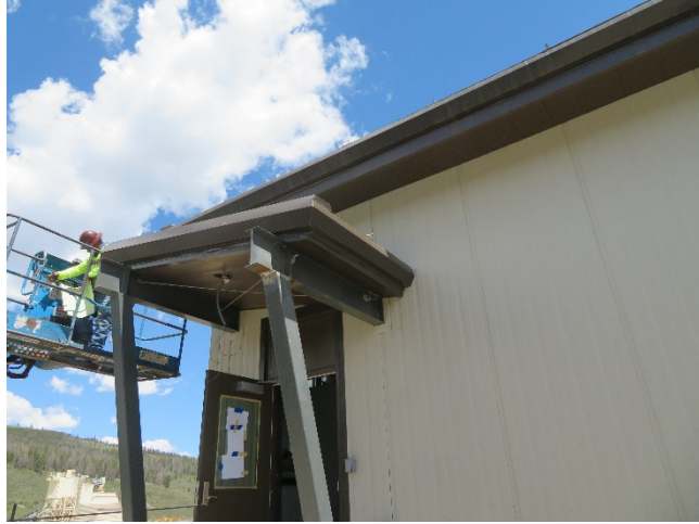
06/05/2020 - Finish Water Pump Station South Entry Canopy Roof
