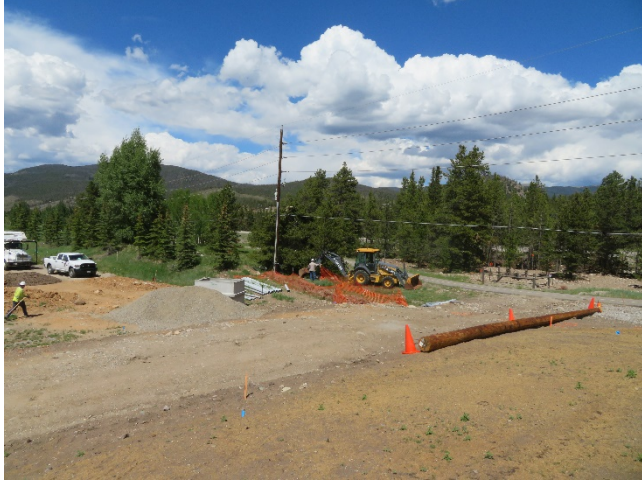
6/23/2020 - Sturgeon Electric Relocation of Overhead Power to Underground
