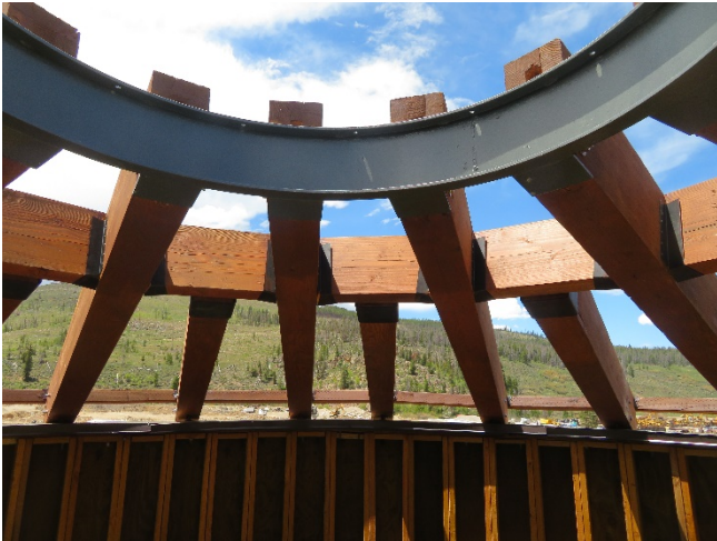
06/01/2020 – Blend Tank Roof
