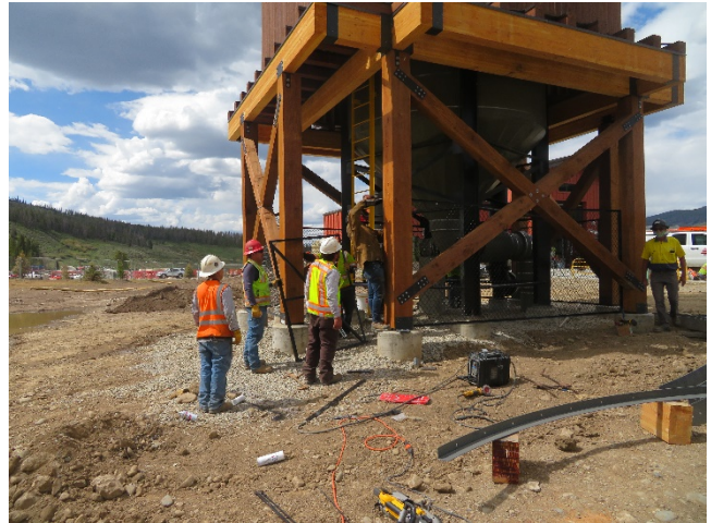
06/02/2020 – Blend Tank Fence
