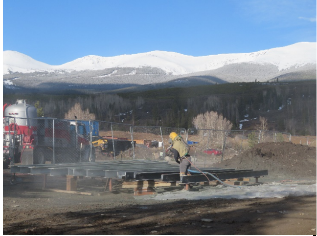
05/12/2020 – Administration Building South Canopy Roof Steel Sand Blasting
