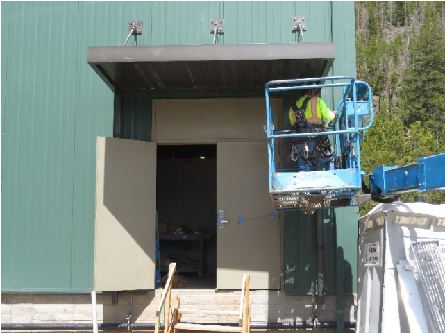
05/07/2020 – Raw Water Pump Station West Entry Canopy
