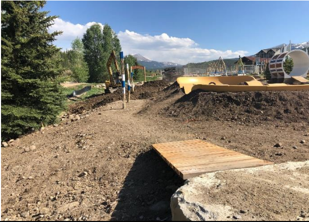
Construction of the "strider" bike park.
