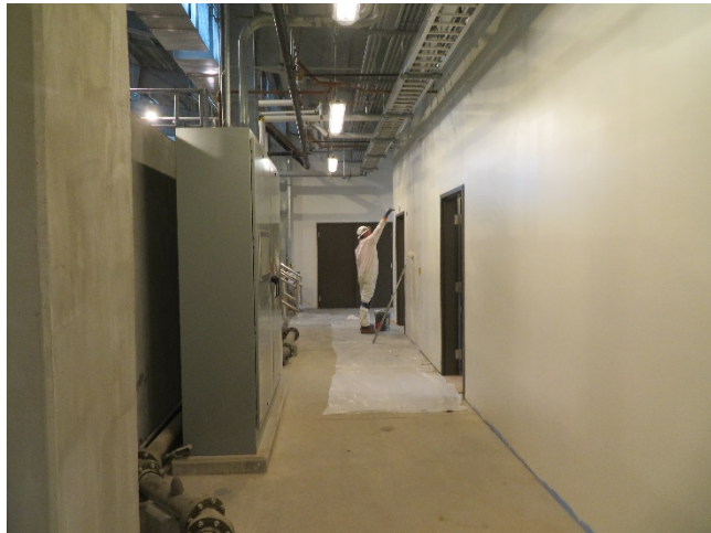
05/15/2020 – Main Treatment Building Wall Painting
