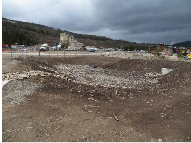
05/11/2020 - Storm Water Detention Pond
