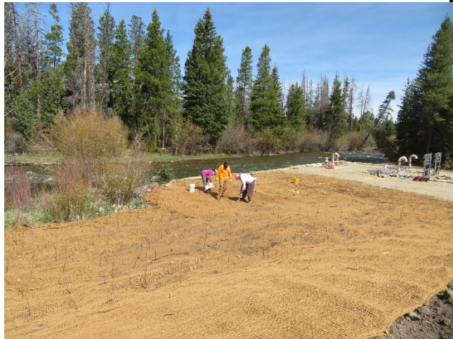
05/18/2020 – Raw Water Pump Station Wetlands Restoration
