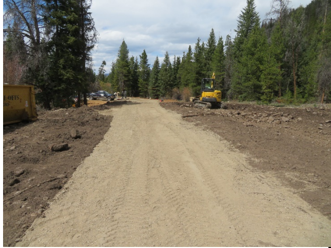
05/14/2020 – Road Base Road to Inlet Structure
