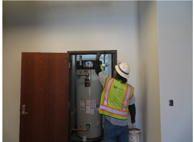
05/08/2020 Administration Building Painting Hollow Metal Jambs
