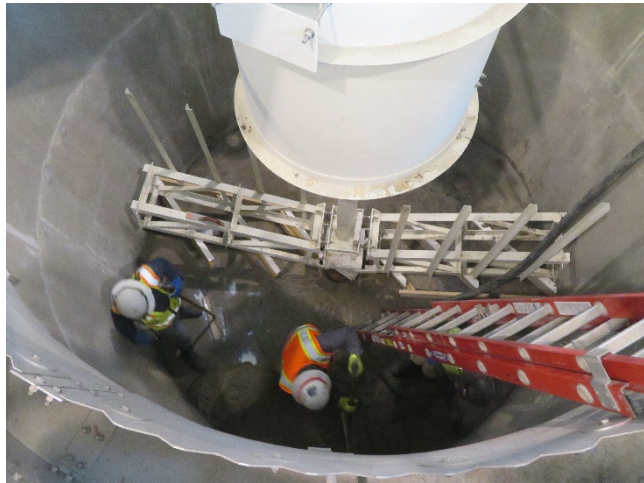
05/12/2020 – Residuals Gravity Thickener Grouting
