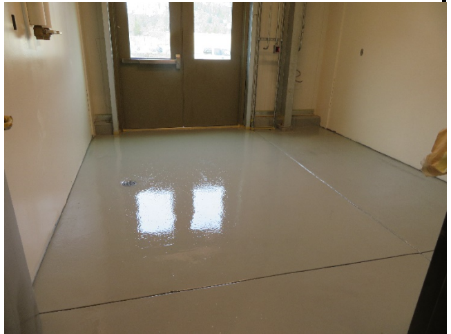
04/23/2020 – MTB Future Chemical Room Floor Epoxy
