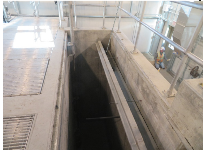
04/29/2020 – Sedimentation basin Influent Weir
