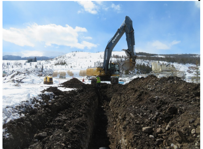
04/14/2020 – Storm Water Line A
