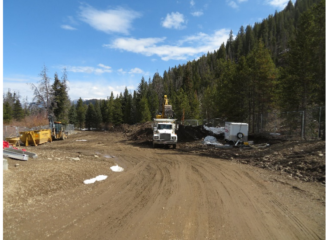
04/22/2020 – Raw Water pump Station Exporting Top Soil
