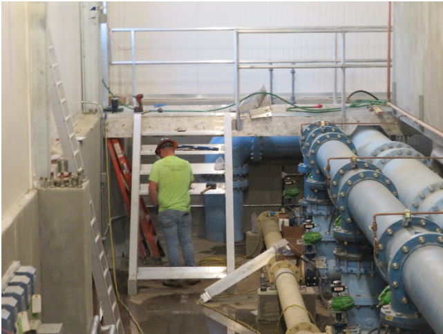
04/01/2020 – Filter Pipe Gallery Elevated Walkway Stair
