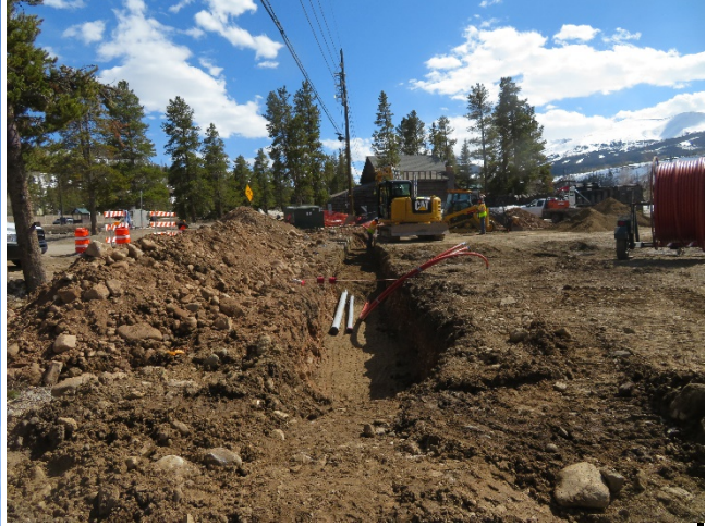
04/27/2020 – Overhead Power reroute Underground
