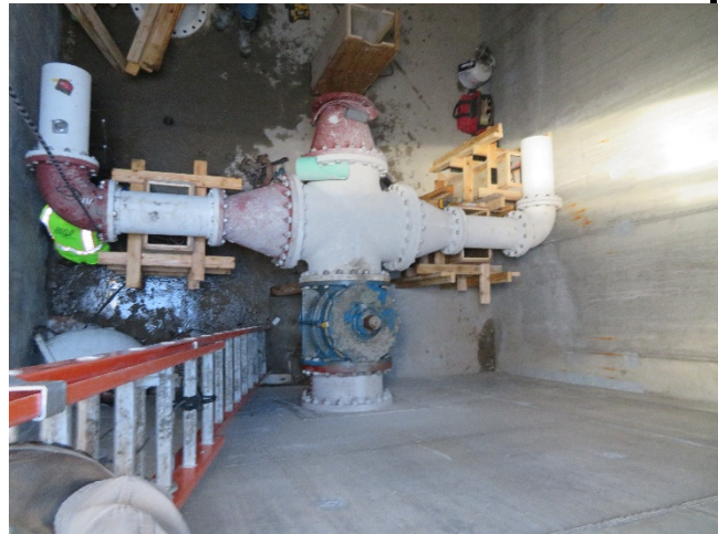
04/20/2020 – Backwash Waste Tanks Pipe Supports
