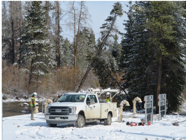
04/14/2020 – Low Lift Pump Station Town of Breckenridge Submersible Pump Training
