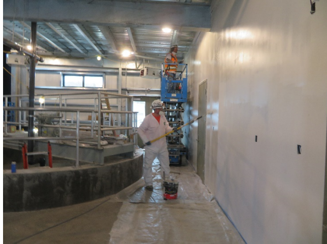
04/15/2020 - Residuals Painting Drywall
