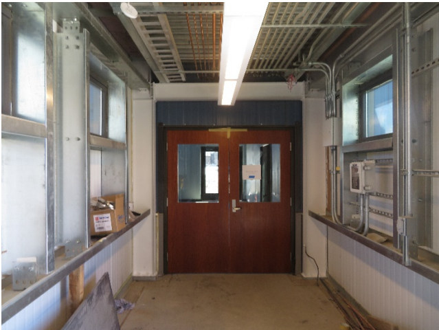
04/08/2020 – Covered Walkway Structural Steel Painted
