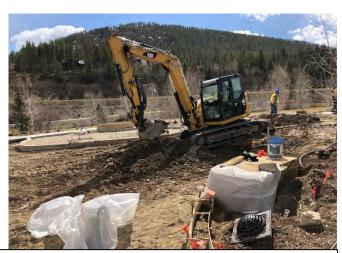
Excavation, grading, concrete curbing, and placement of boulders was completed this week for the new play areas. The area shown above will have custom "nature play" features installed in the coming weeks.
