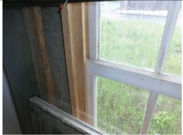
Figure 24: Interior of the Room 2 sashes.
