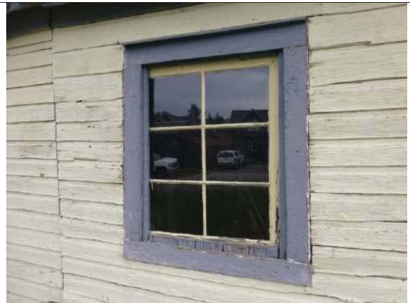
Figure 22: South façade, fixed sash in the Shed room.
