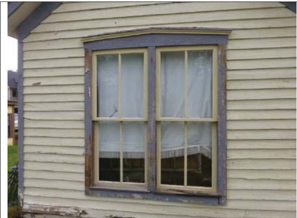
Figure 21: Pair of double hung windows in the west façade.
