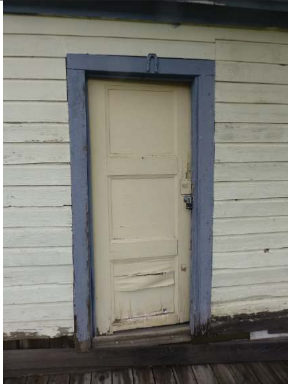
Figure 18: 3-panel main entry door.
