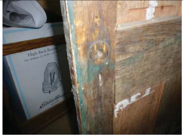
Figure 19: 4-panel door between Room 2 and the Shed.
