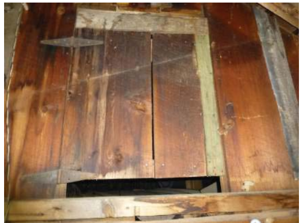
Figure 20: Plank attic access door at the Shed.
